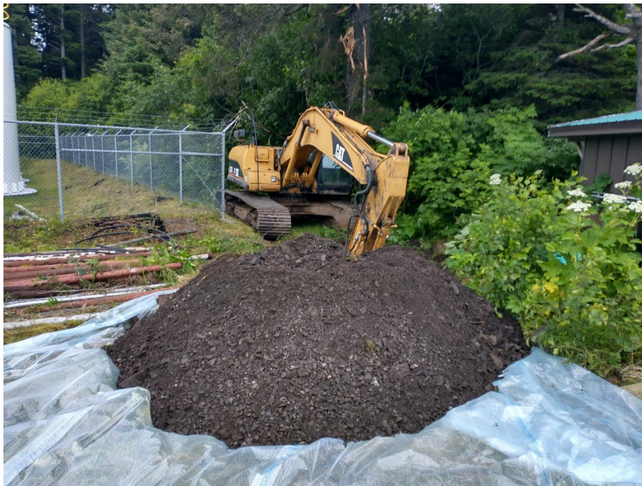
Photo 3: Excavating Test Pit TP1, view southwest. (July 19, 2023)
