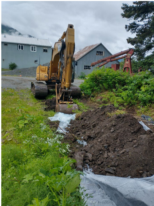
Photo 5: Excavating Test Pit TP5, view east. (July 19, 2023)
