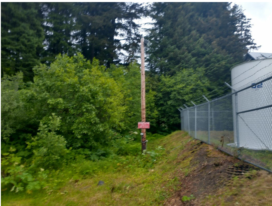
Photo 2: Location of proposed sewer alignment on the south side of the tank farm, view west. (July 19, 2023)
