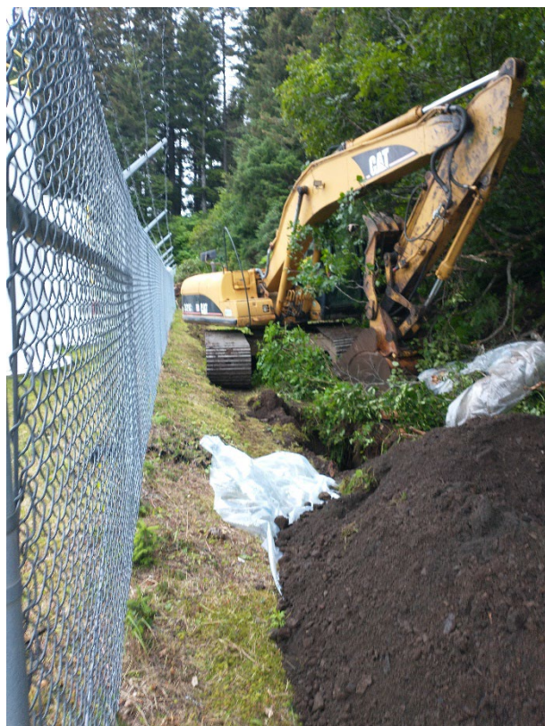
Photo 6: Excavating Test Pit TP6, view south. (July 19, 2023)
