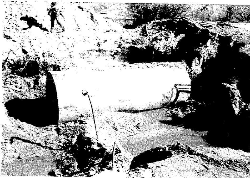
Photo 4: Tank No. 3, a 4,000-gallon UST, in place in the excavation.
