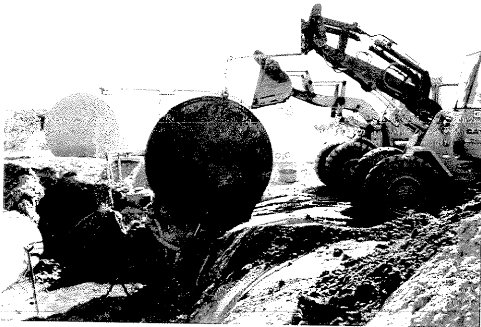
Photo 2: Tank No. 2 during removal.
