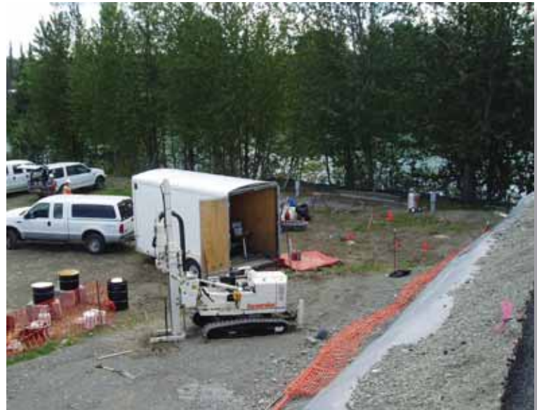
Improper disposal of dry cleaning fluids was a significant source of contamination before strict hazardous waste laws took effect. Small amounts of its hazardous components are highly toxic and don't break down easily. This cleanup of a former dry cleaner next to the Kenai River has involved treating contaminated surface soil at the site, and innovative underground injections (shown) of hydrogen-releasing compounds to speed decomposition of tetrachlorethene and its "daughter products" in subsurface soil. The Kenai River is visible through the trees. DEC photo.
