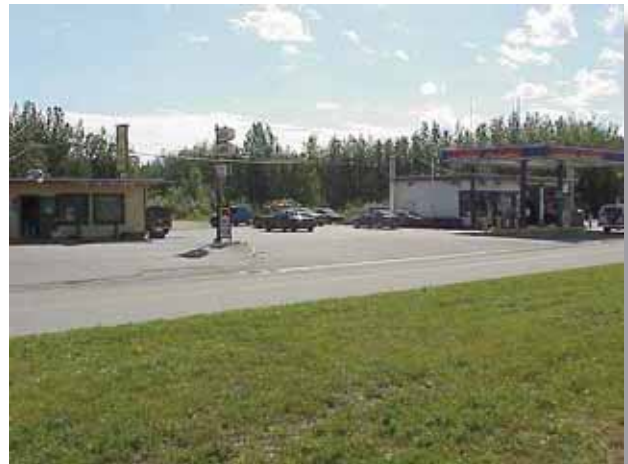
Laws passed in the 1980s and 1990s acknowledged that leaks from gas stations were the sources of a great deal of underground contaminated soil and groundwater, sometimes contaminating drinking water. (DEC photo)
