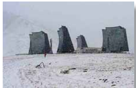
These “White Alice” antennae on St. Lawrence Island are similar to others across Alaska. They served as part of a system of military/civilian communication system across Alaska from 1956 to 1979.
