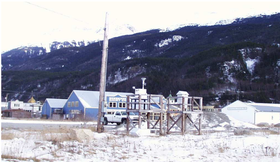
Figure 3: PM 2.5 monitoring site operated by the Skagway Tribal Council
