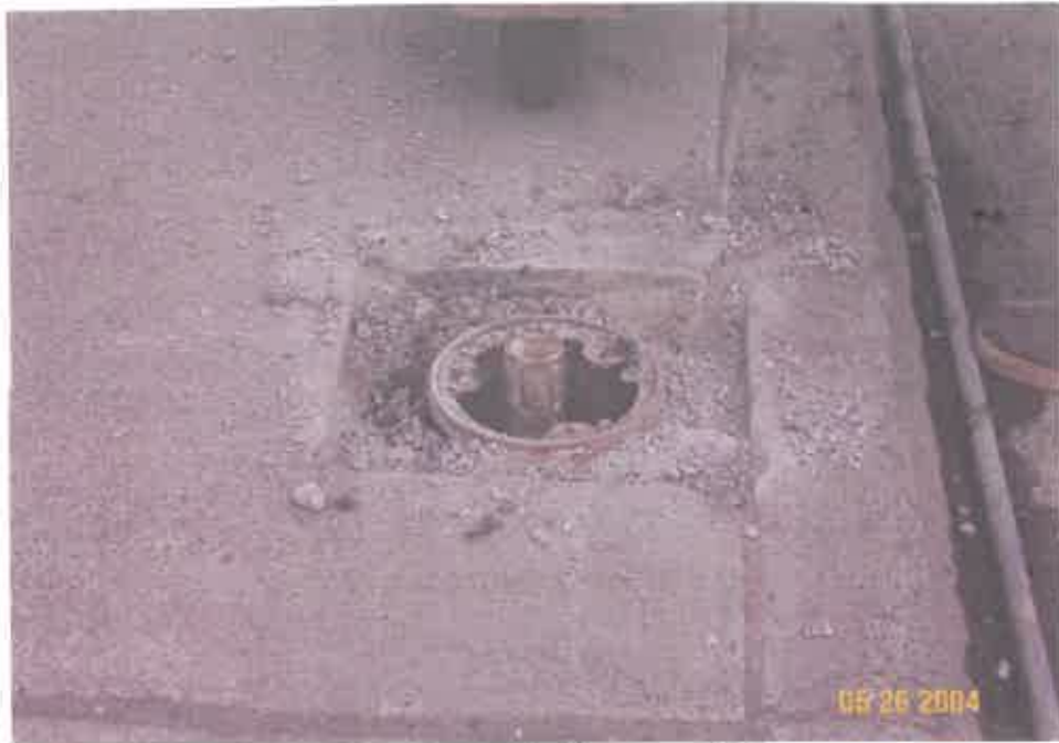
After concrete around security casing was jackhammered. Riser extension is visible.
