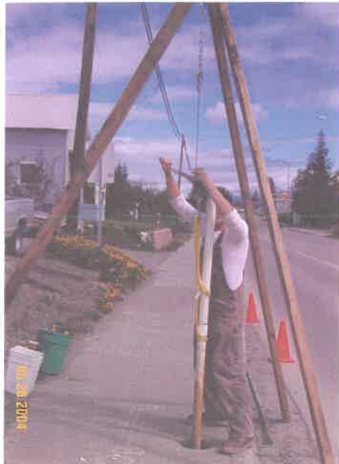
Typical tripod set up (MW2); hoisting well pipe from borehole.
