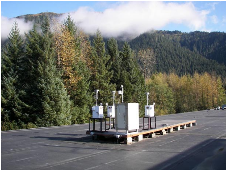
DEC air quality monitoring equipment at Floyd Dryden Middle School in the Mendenhall Valley.
