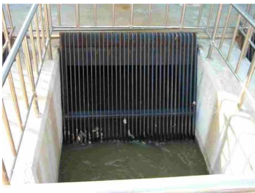
Manually cleaned bar screen
