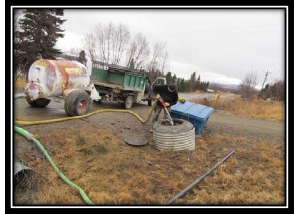
Paul Arne, BBAHC RMW, assists with sewer manhole flushing in Nondalton.
