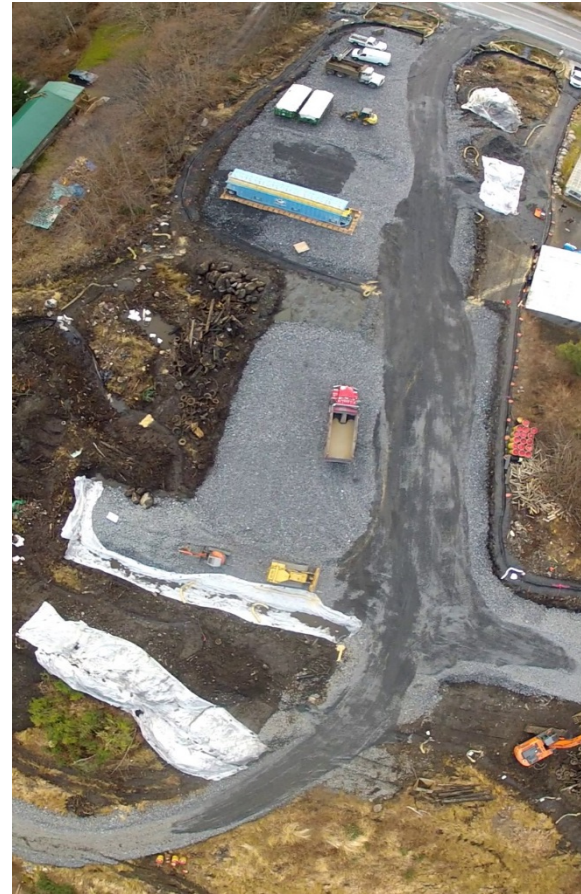
Access Road and Equipment Pads Constructed
