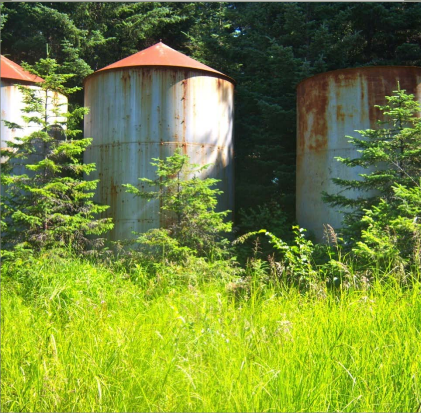
Abandoned fuel tanks
