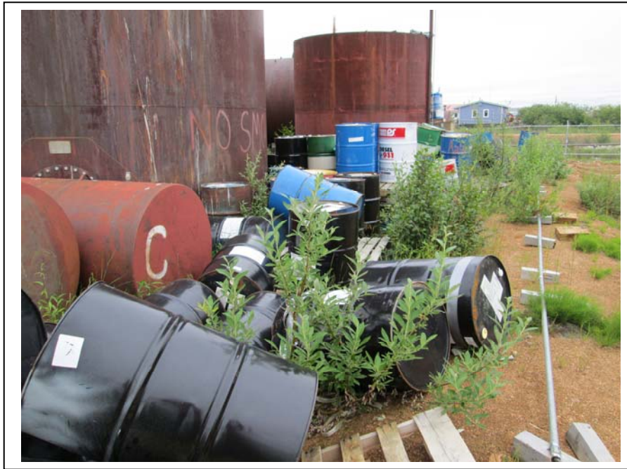
Photo 9: Looking north, numerous drums were stored within the Old Tank Farm berms. Some of the drums stored upright in the background contained liquid. (July 18, 2012)
