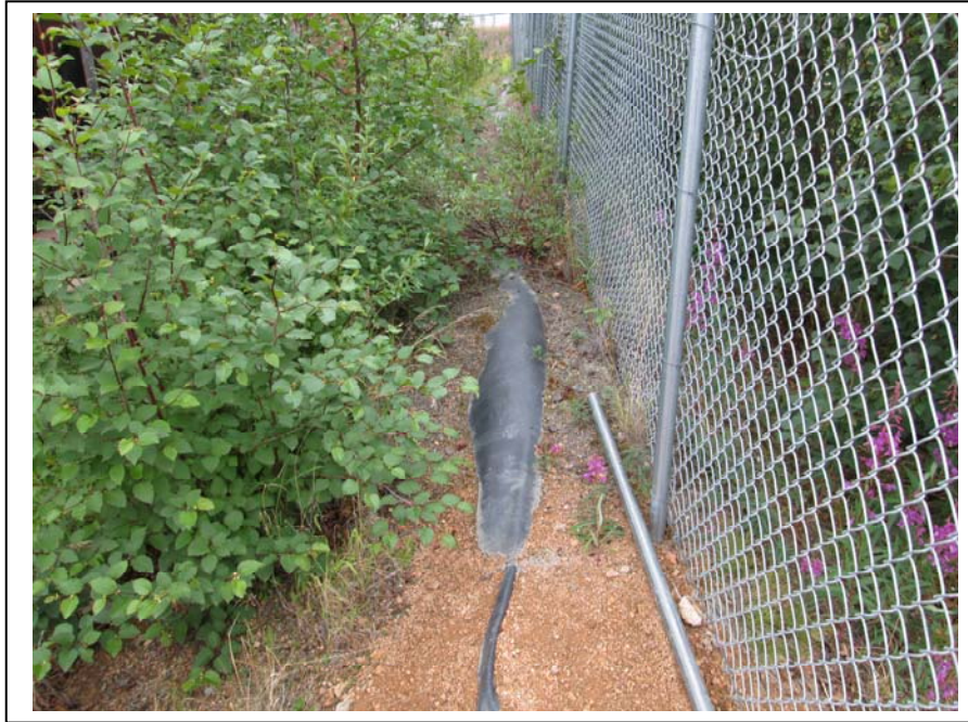
Photo 7: Looking west along the northern fence of the Old Tank Farm. Black liner was observed along the northern berm of the Old Tank Farm. (July 18, 2012)
