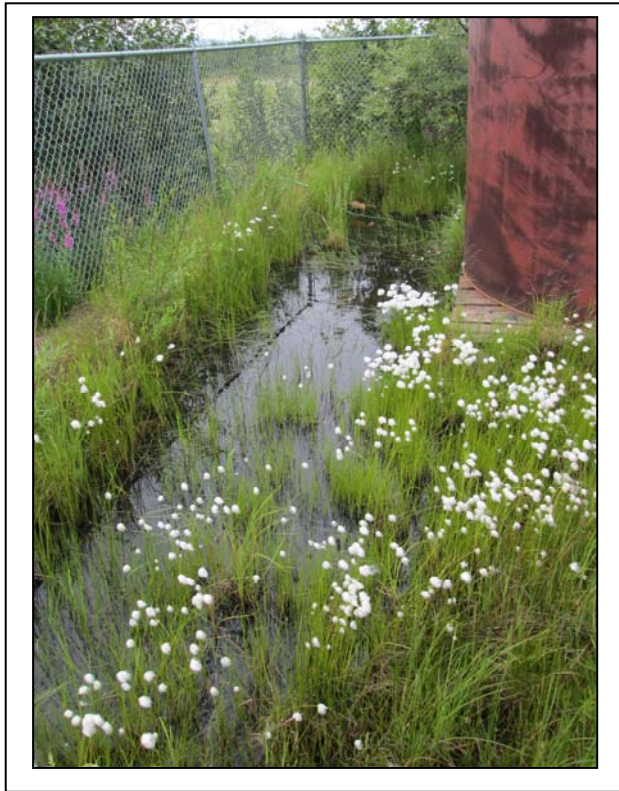
Photo 5: Looking west, ponded water was observed within the bermed area of the Old Tank Farm. No hydrocarbon odor or sheen was observed at the time of our site visit. (July 18, 2012)
