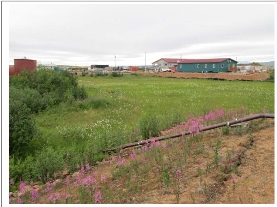
Photo 11: Looking southeast toward the Property from the New Tank Farm. The Summit Camp Building (blue) is present in the upper right hand corner of the photo. (July 18, 2012)
