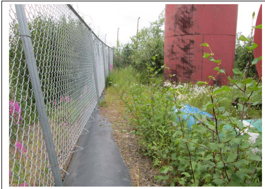
Photo 6: Looking west along the southern fence of the Old Tank Farm. Black liner was observed along the top of the southern berm. (July 18, 2012)
