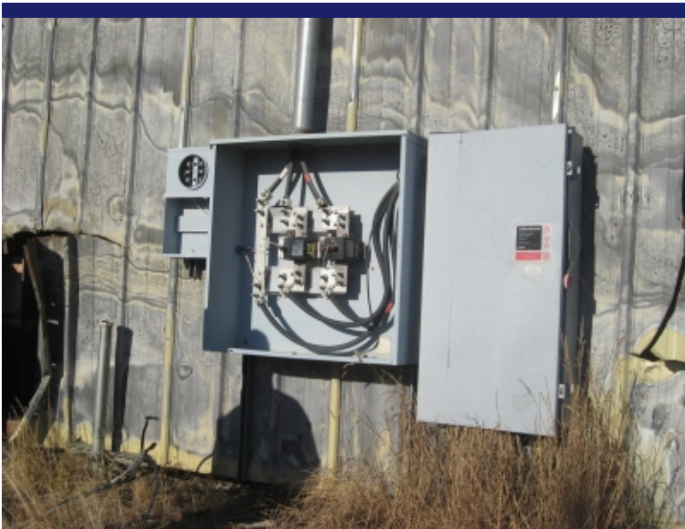
Photo 11 Exterior electrical box on southern end of building.
