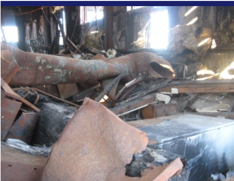
Photo 3 Interior of burned community center facing west.
