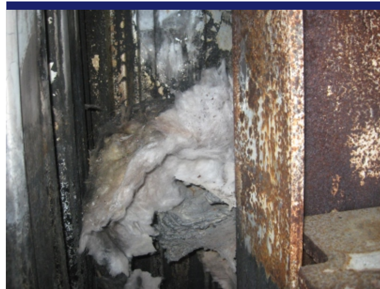
Photo 8 Burned wall insulation.
