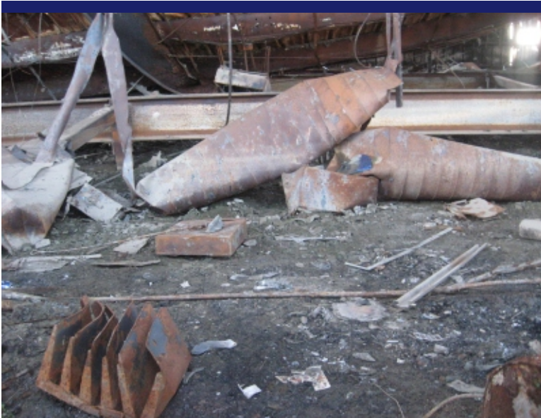
Photo 5 Interior of building showing exposed dirt.
