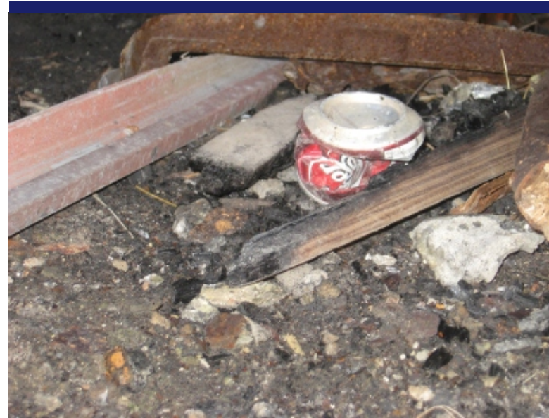
Photo 14 Under the southwest end of the building.
