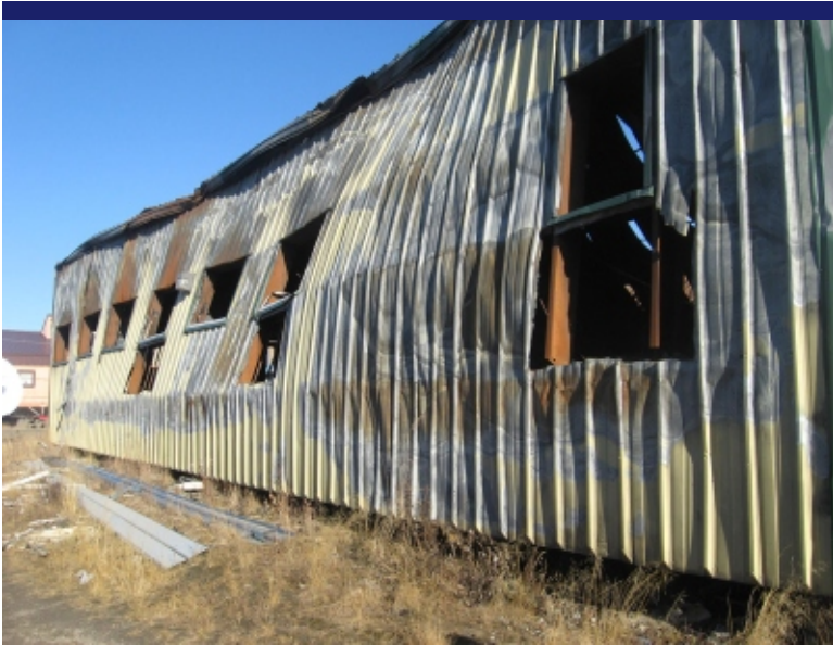
Photo 13 West side of building.
