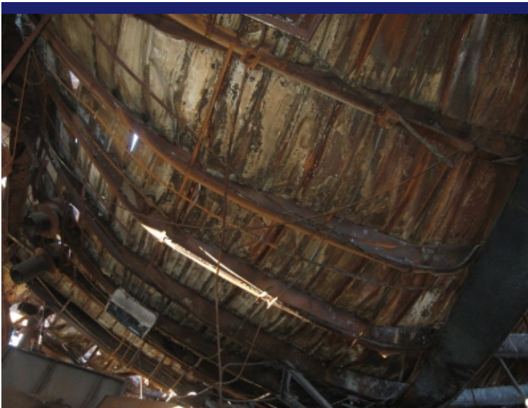
Photo 7 Remaining, metal ceiling. All insulation is gone from the ceiling.
