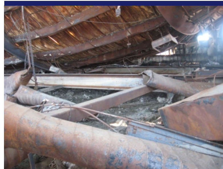
Photo 4 Interior of burned community center facing west showing dirt exposed after the floor burned.
