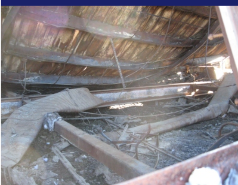
Photo 17 Interior of the building pictured from the west side.
