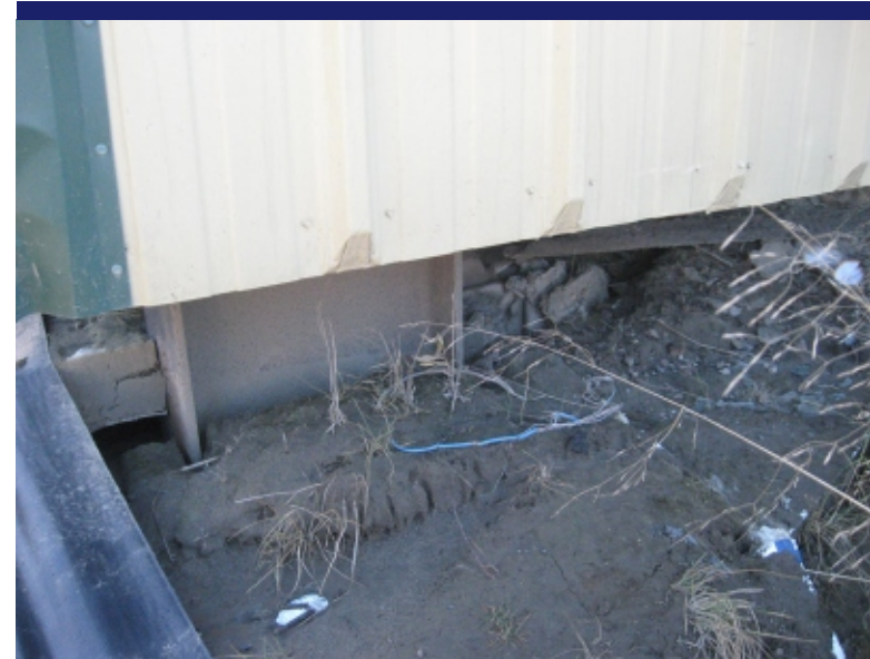
Photo 2 Corner post under community center.
