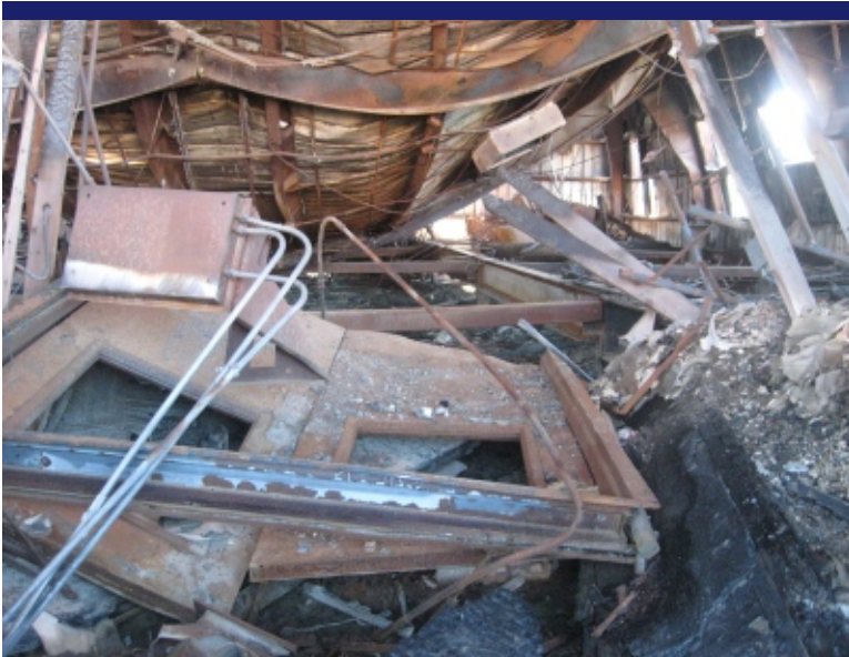
Photo 1 Interior of burned community center.
