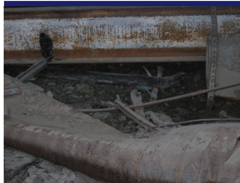
Photo 16 Interior of the building pictured from the west side.
