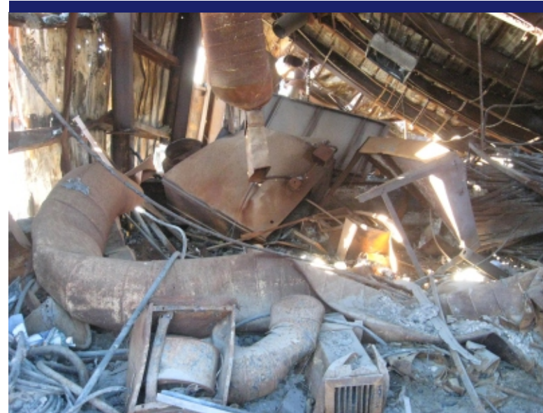
Photo 6 South end of building interior. Large, square metal frames are the remains of the building's furnace which prior to the fire was on the second level.
