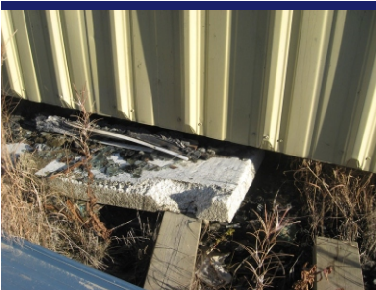
Photo 15 Styrofoam under the west end of the building used to help level the foundation.
