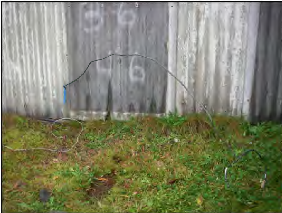
PHOTOGRAPH 42: WIRES PROTRUDING FROM BACK OF BUILDING.
