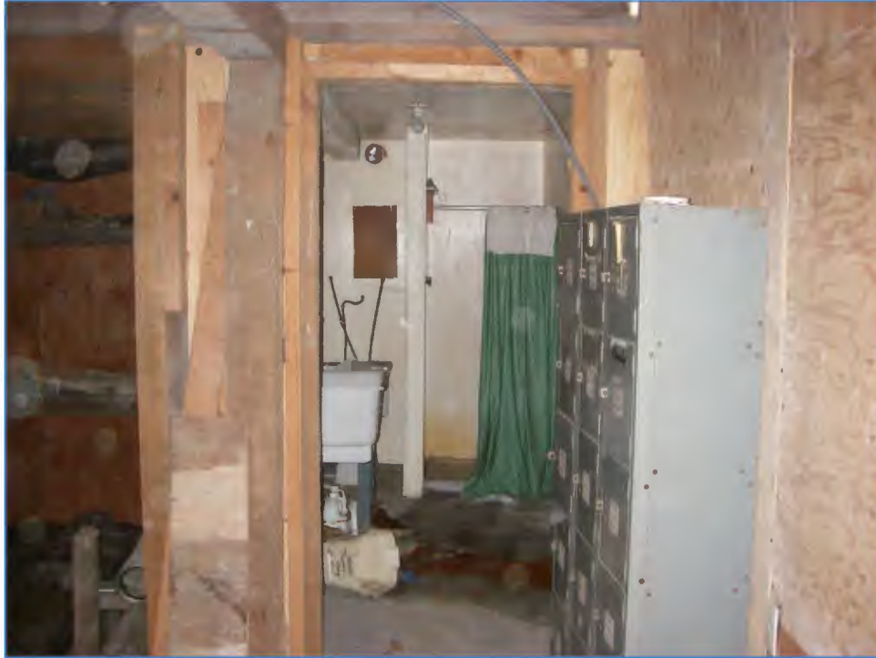
PHOTOGRAPH 4: BATHROOM ON FIRST FLOOR, BACK RIGHT OF BUILDING.
