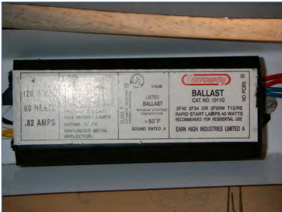
PHOTOGRAPH 10: FLUORESCENT LIGHT BALLAST IN LOFT.
