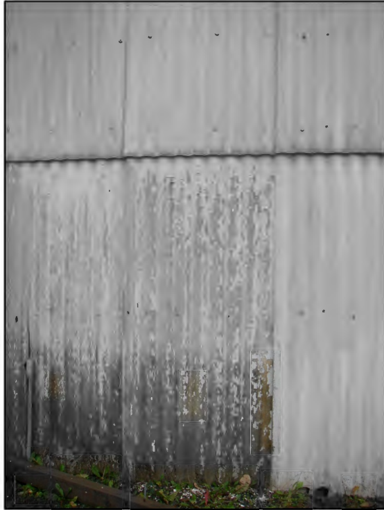
PHOTOGRAPH 35: ZOOMED-OUT VIEW OF EXTERIOR SEEN IN PHOTOGRAPH 34; PAINT CHIPPING IS HEAVIER IN SOME SIDING VERSUS OTHERS.
