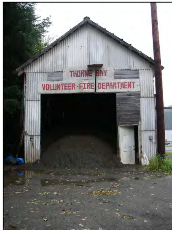
PHOTOGRAPH 54: FRONT VIEW OF OLD FIRE HALL; BLUE TARPS VISIBLE ON LEFT SIDE OF BUILDING.
