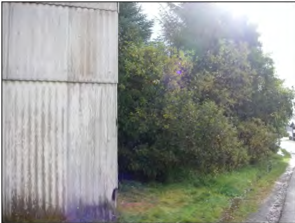
PHOTOGRAPH 38: NORTH CORNER OF BUILDING.
