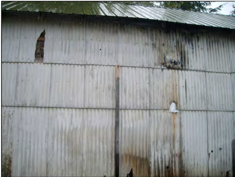
PHOTOGRAPH 64: EXTERIOR RIGHT SIDE OF BUILDING.
