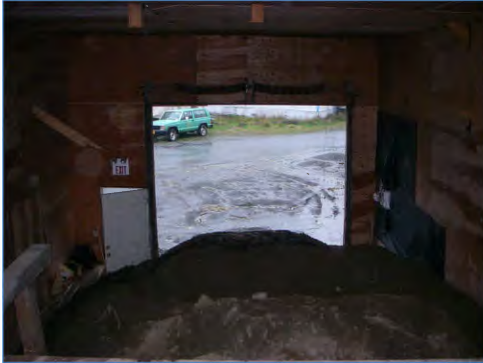
PHOTOGRAPH 6: VIEW FROM LOFT LOOKING OUT OF BUILDING.
