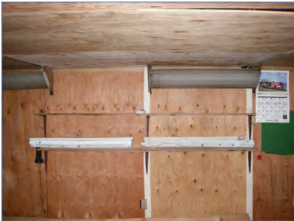
PHOTOGRAPH 5: FLUORESCENT LIGHT FIXTURES IN LOFT.
