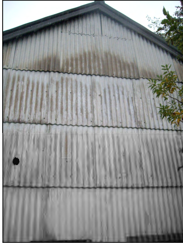
PHOTOGRAPH 65: EXTERIOR BACK OF BUILDING.
