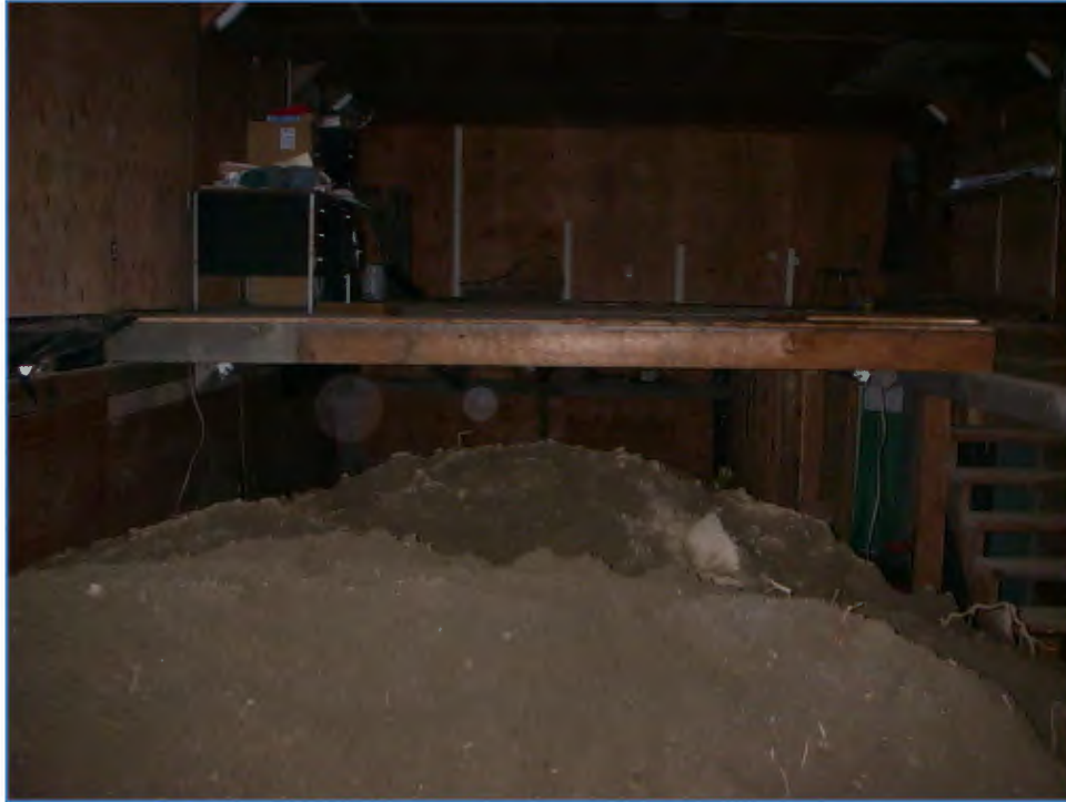
PHOTOGRAPH 19: INTERIOR VIEW OF SAND PILED UP TO LOFT, LOOKING FROM FRONT OF BUILDING TO THE BACK. SIMILAR VANTAGE POINT AS PHOTOGRAPHS 1 AND 2.
