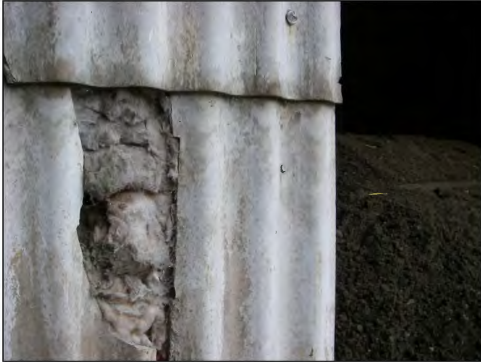
PHOTOGRAPH 53: APPEARS TO BE FIBERGLASS INSULATION EXPOSED ON FRONT OF BUILDING WHERE CEMENT SIDING HAS BROKEN OFF.
