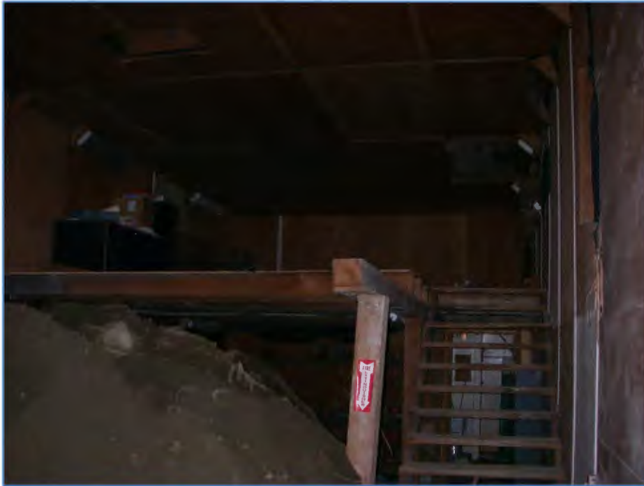
PHOTOGRAPH 1: INTERIOR VIEW OF SAND PILED UP TO LOFT, LOOKING INTO BUILDING.
