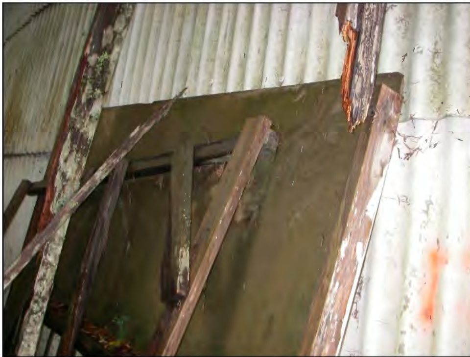
PHOTOGRAPH 48: WOOD LEANING ON LEFT SIDE OF BUILDING.
