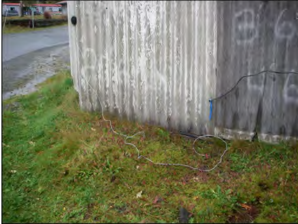
PHOTOGRAPH 43: WIRES PROTRUDING FROM BACK OF BUILDING (EXTERIOR).
