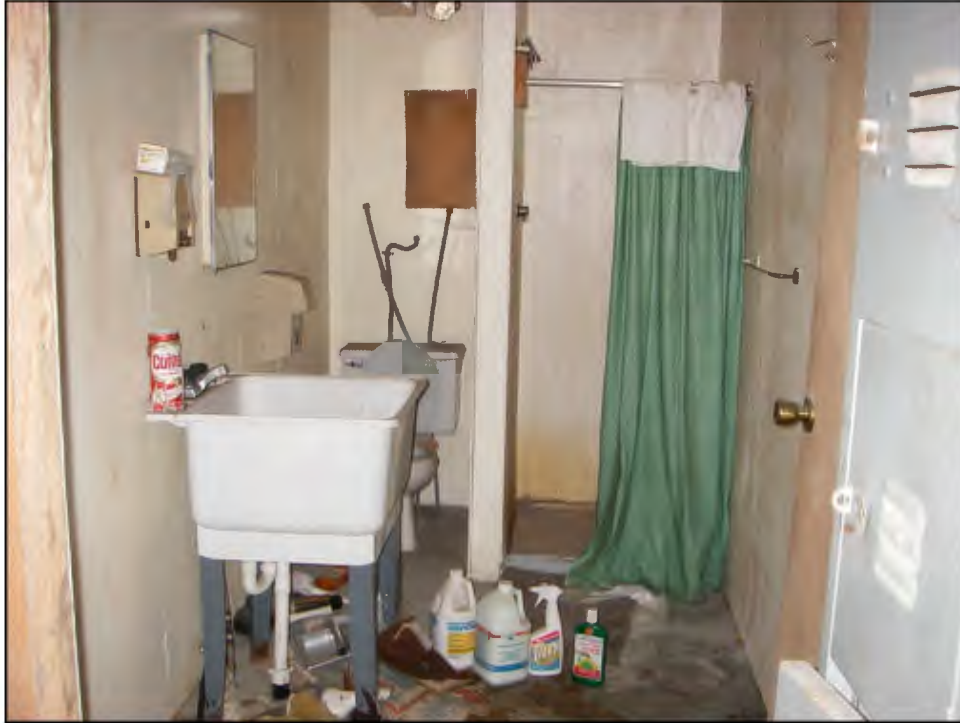
PHOTOGRAPH 27: LOCKERS AND BATHROOM.
