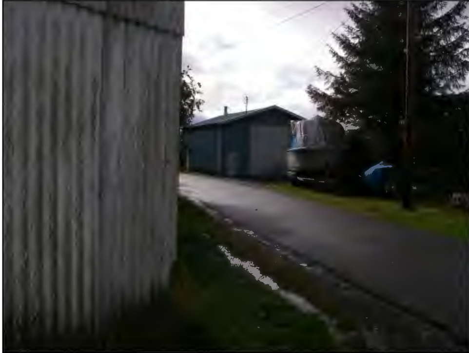
PHOTOGRAPH 39: BACK (EXTERIOR) OF BUILDING.
