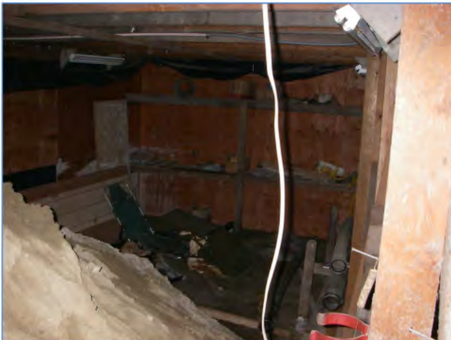
PHOTOGRAPH 3: BACK PORTION OF FIRST FLOOR; ONLY AREA ON FIRST FLOOR NOT COVERED IN SAND.
