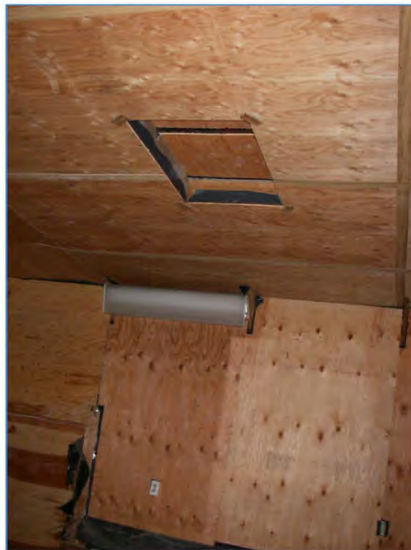
PHOTOGRAPH 18: VIEW OF CEILING AND APPARENT ATTIC ENTRY FROM LOFT.
