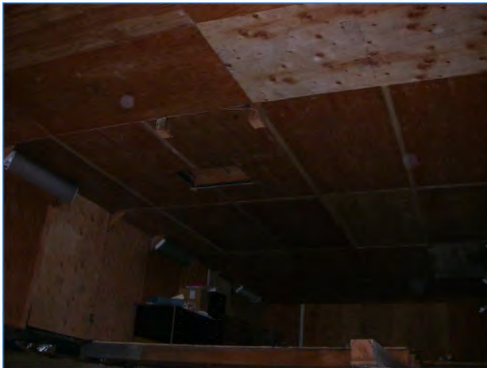
PHOTOGRAPH 20: VIEW FROM FIRST FLOOR LOOKING UP TO LOFT AND APPARENT ATTIC ENTRY IN CEILING.
