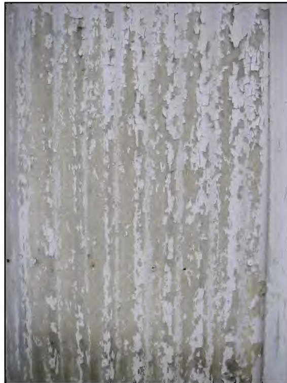
PHOTOGRAPH 34: EXTERIOR OF BUILDING; SIDING IS GENERALLY INTACT, BUT THE PAINT IS CHIPPING.
