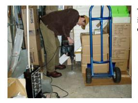
The first step is to drill a 1-inch diameter hole 3 inches into the foundation, followed by a 3/8-inch diameter hole the rest of the way through the slab.
