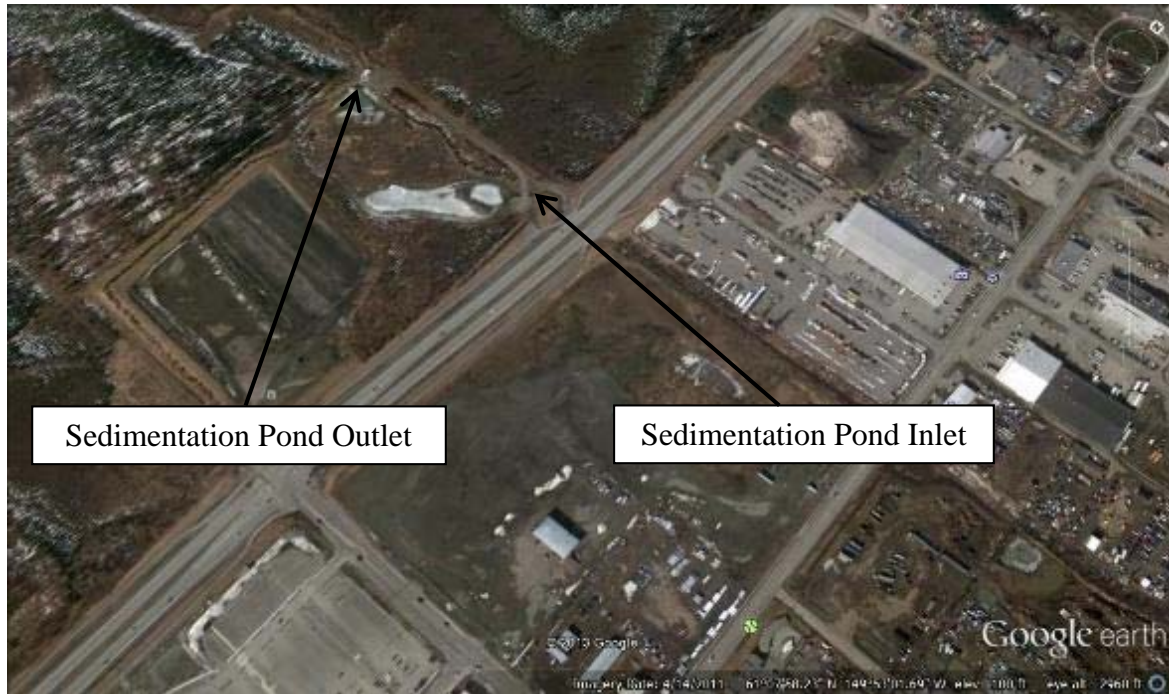
Photograph 2. Aerial view of snow storage and sedimentation pond west of C Street.
