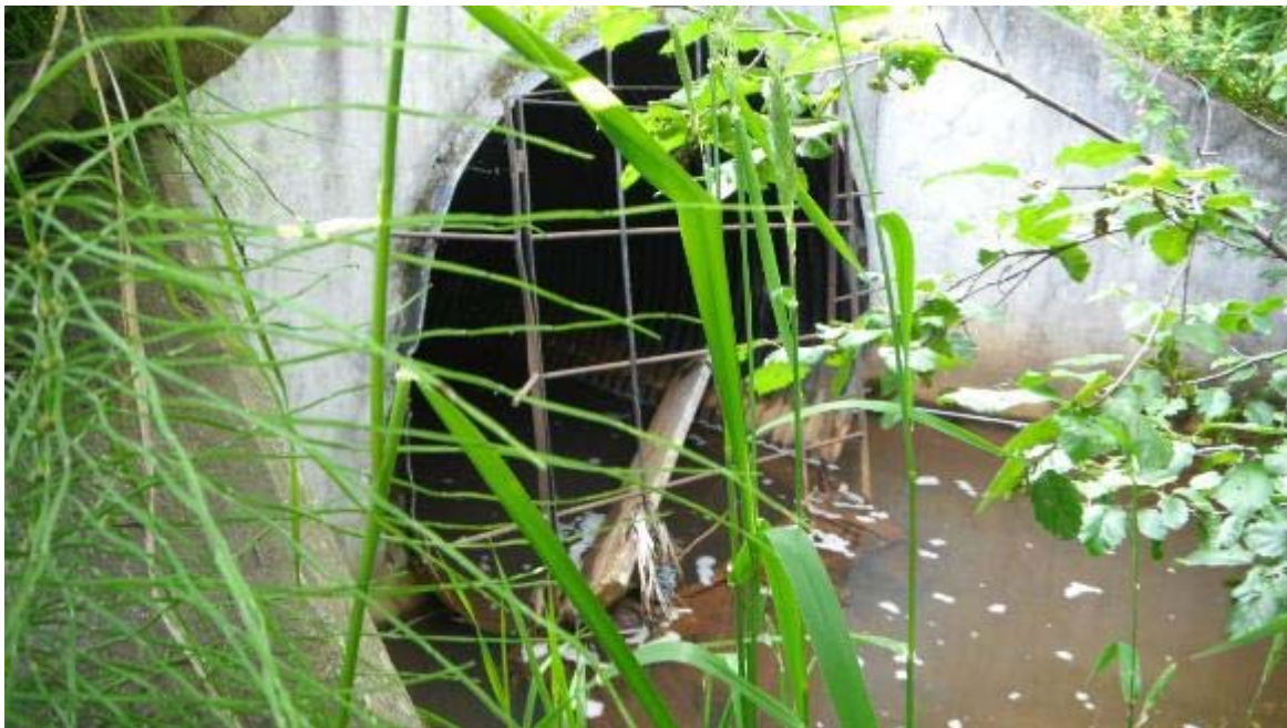
Photograph 7. Downstream culvert outlet at Victor Road on July 19, 2013.
