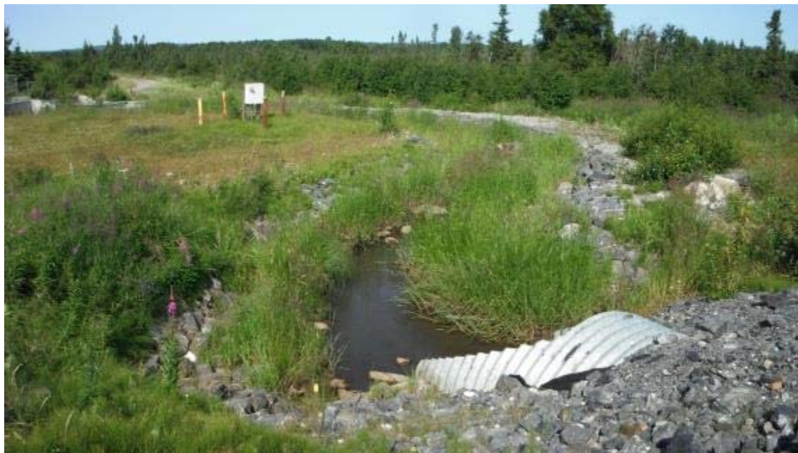
Photograph 3. Campbell Lake tributary where it exits from the C Street culvert on July 19, 2012.
