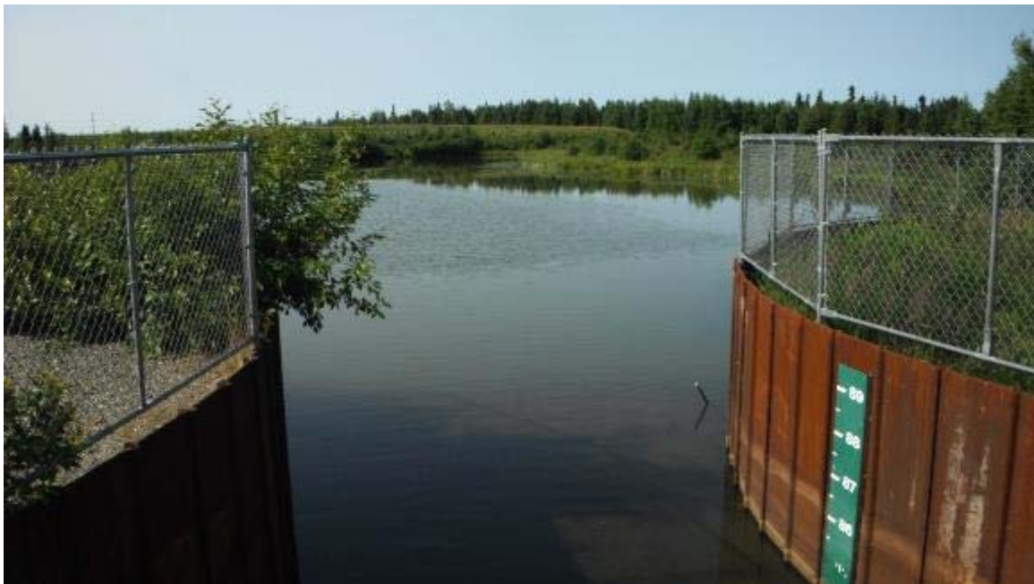
Photograph 5. Inlet to the C street sedimentation pond on July 19, 2012.
