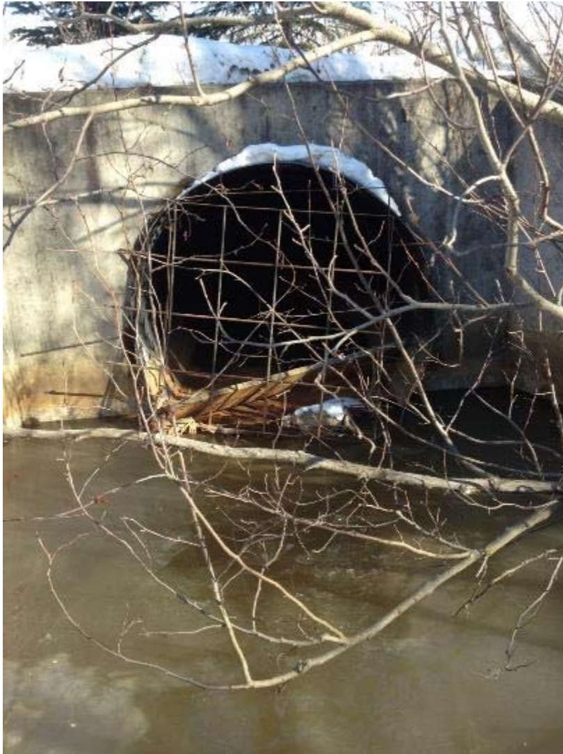
Photograph 21. Ice surface at Victor Road culvert on March 19, 2013.
