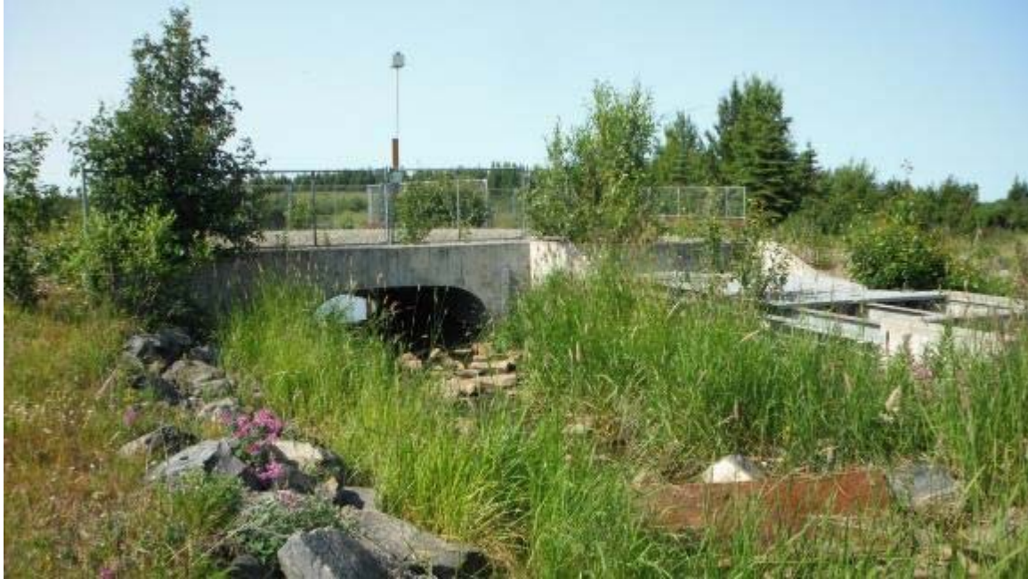
Photograph 4. Inlet to sedimentation pond July 19, 2012.
