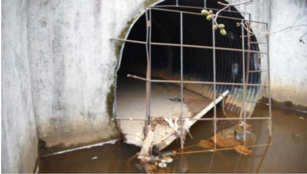
Photograph 19. Foam and debris at Victor Road culvert outlet on September 27, 2012. Turbidity was 10.4 NTU.
