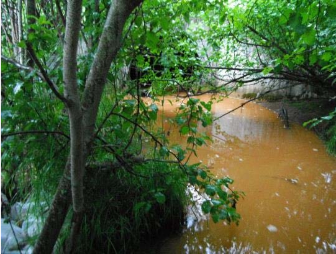
Photograph 13. Outlet of Victor Road Culvert on August 16, 2012. Turbidity was 183 NTU.
