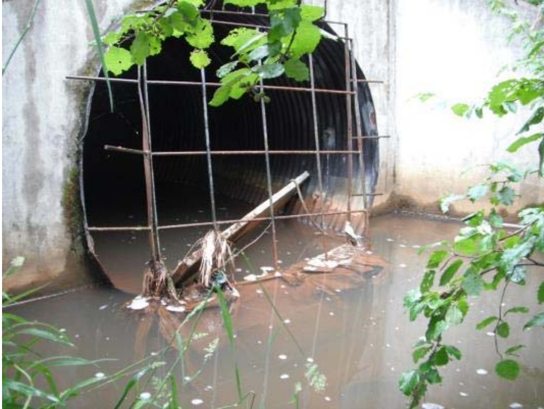
Photograph 12. Outlet of Victor Road culvert on August 1, 2012. Turbidity was 9.51 NTU.
