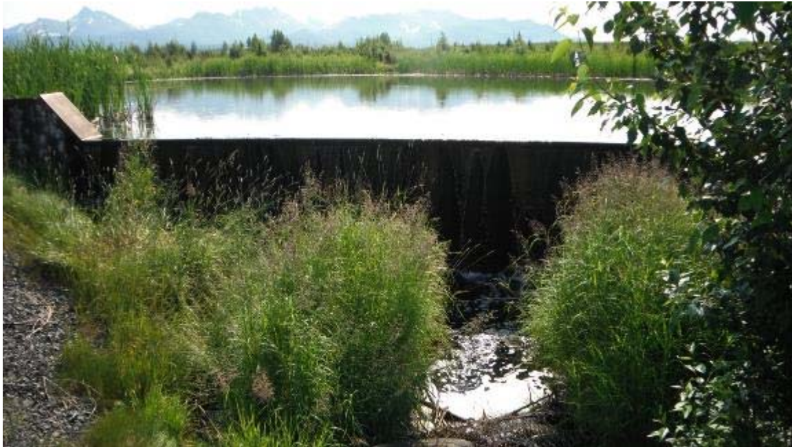
Photograph 6. Outlet C street sedimentation pond spillway on July 19, 2012. Campbell Lake tributary enters a culvert at this location and reemerges on the west side of Victor Road.
