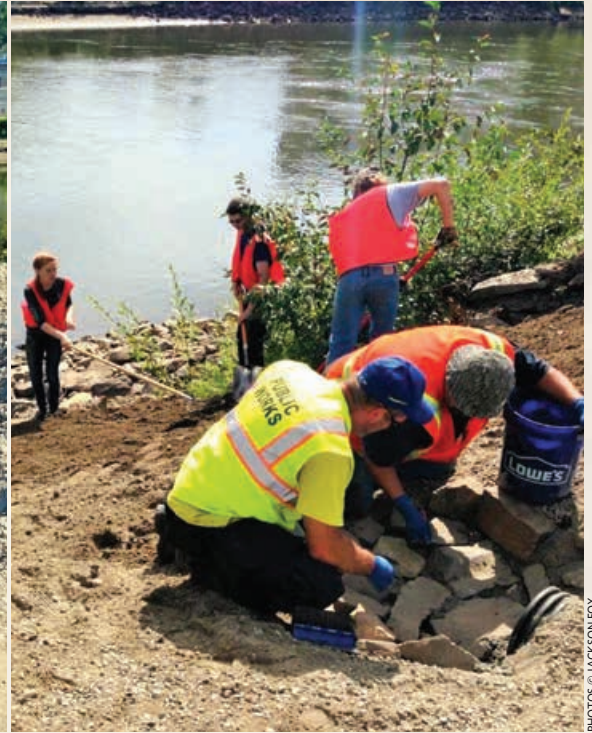
With the concrete chute removed, volunteers worked diligently to rehabilitate the river bank with topsoil, grass seed and live willows.
