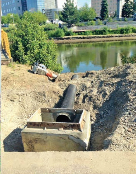
The city installed this catch basin to receive the runoff and capture some of the sediment and litter before spilling the water down the newly vegetated bank.
