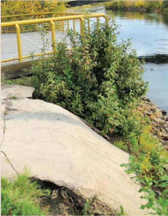
Polluted runoff from the 21,000 square-foot parking lot at Gordon Wear Park drained directly into the river via this concrete chute.
