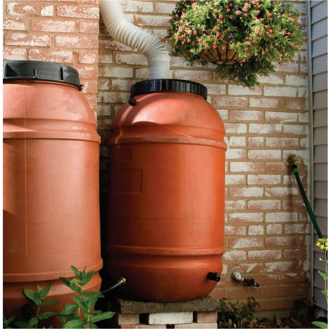
A variety of types of rain barrels are available, from simple garbage cans, wooden, galvanized, ceramic clay or decorative plastic pictured, your needs and budget will determine which is the right application for your project.
