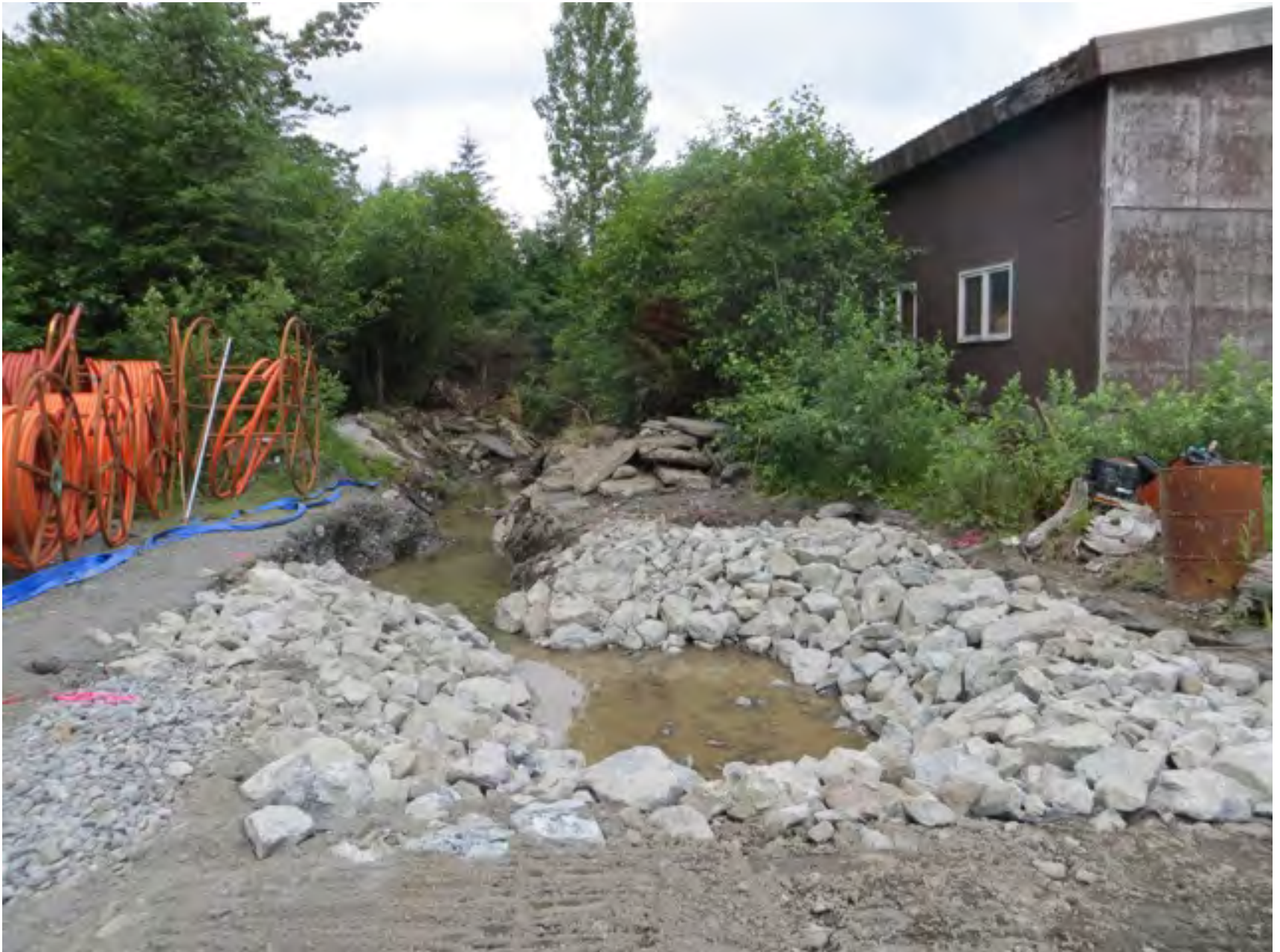
Sediment basin complete
