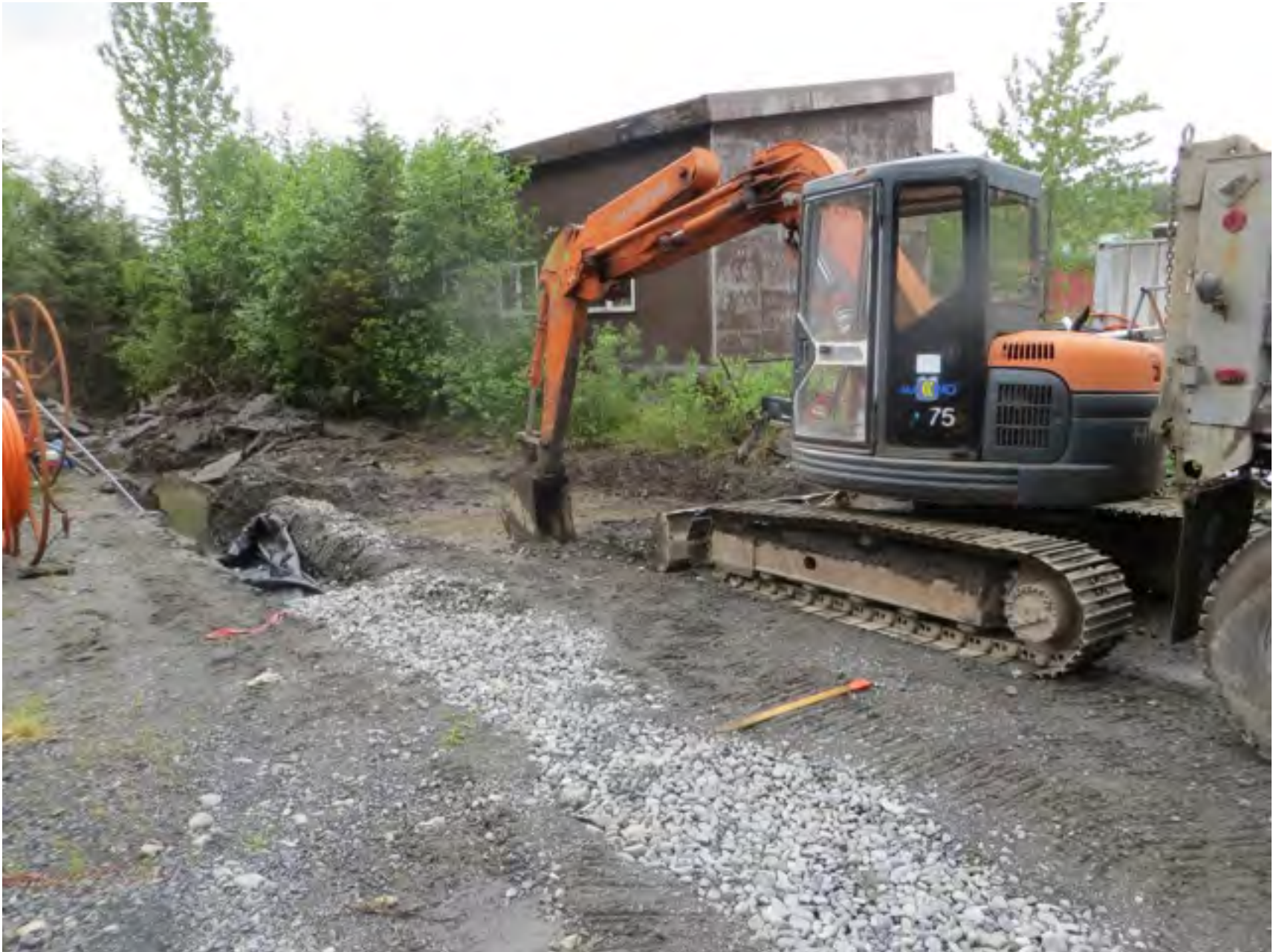
Digging out the sediment basin
