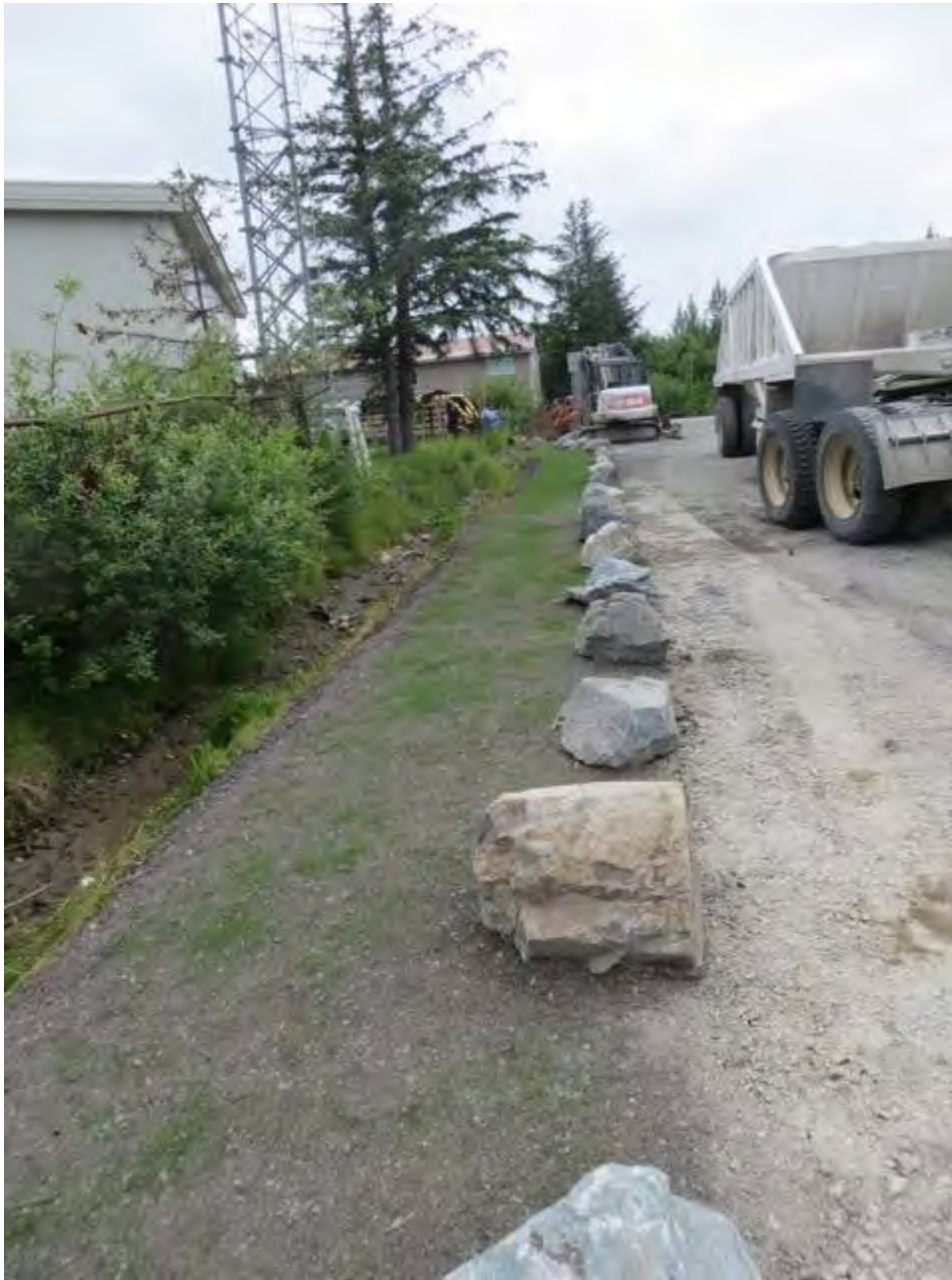
Photos of the buffer on the Wilson lot — grass is sprouting! Those two photos are taken from the same point, looking in two opposite directions (“downstream” and “upstream” on the drainage ditch).
