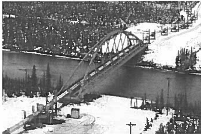
http://tapseis.anl.gov/guide/photo/Gulkana_Bridge.html The pipeline crosses 800 rivers and streams, etc.
