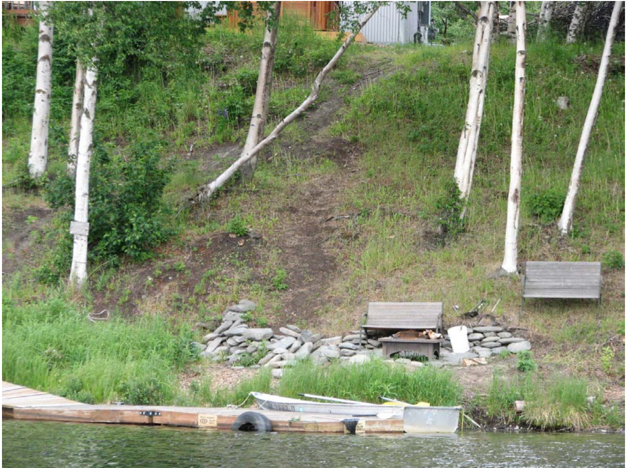
Figure 69. Residential property on the west side of Jewel Lake that received a Poor (C) habitat quality rating, due mainly to the lack of buffer present, bare areas and erosion on a steep slope, and debris (pallets) in the water. (Photo by Dr. Cherie Northon).
