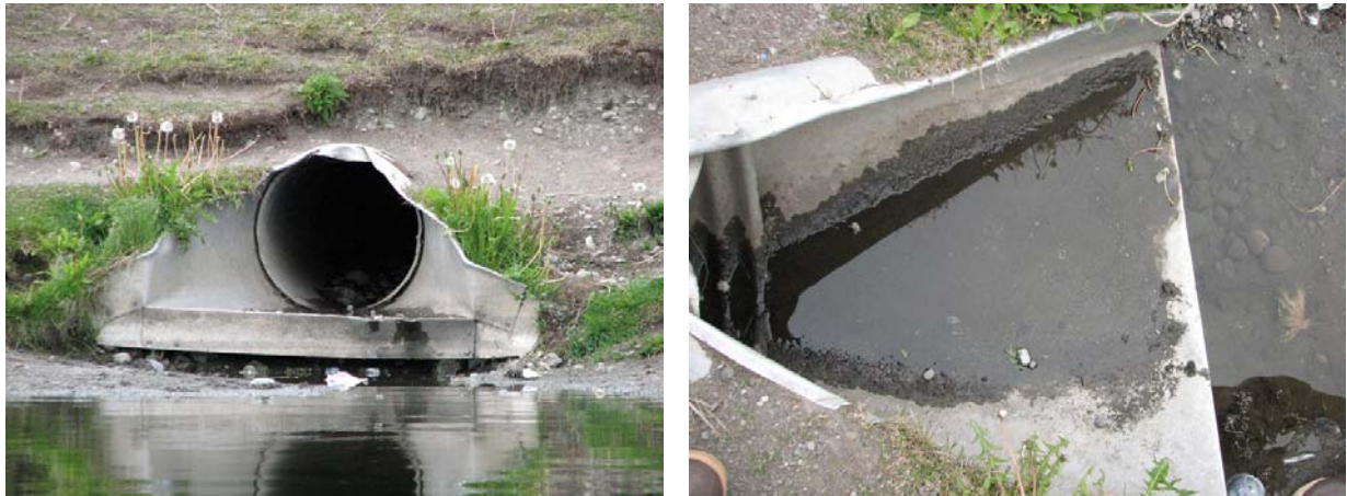
Figure 11. Major stormwater outfall (originates on south side of Dimond Blvd.) after a rain event, June 2010 (Photo by Cherie Northon).
