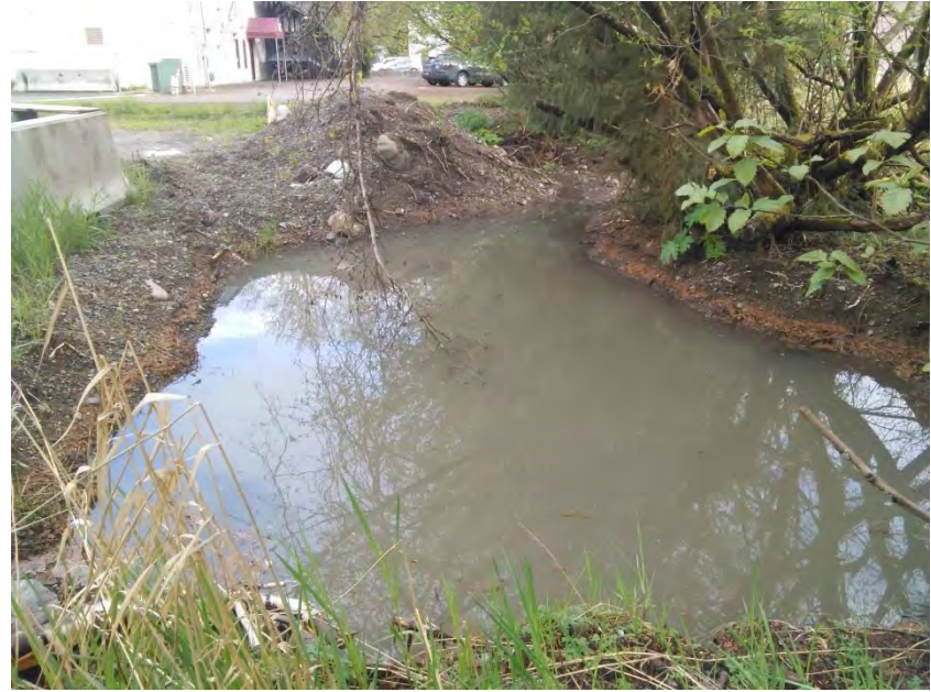
Figure 28. Diversion ditch to divert run off into the excavated hole that will eventually become the rain garden. Photo taken April 2016.
