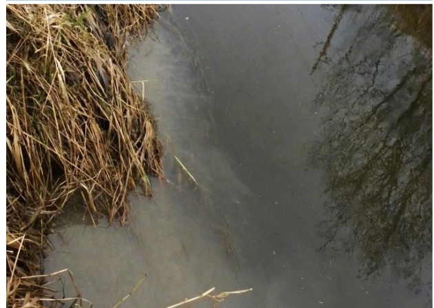
Figure 9. Sediment discharging into Jordan Creek from the Edward K. Thomas building site prior to the installation of the rain garden.
