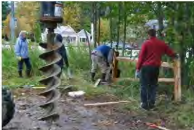
Photo by Angie Flickinger - Volunteers work to install a split rail cedar fence along Jordan Creek. They hope the fence will prevent plowed snow, and its accompanying contaminants, from entering the creek.
