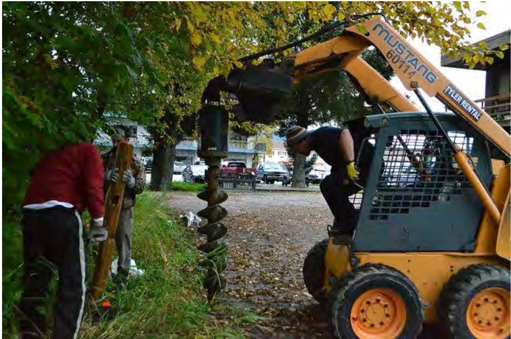
Figure 12. Post-hole digging with an auger. Photos taken September 2015.
