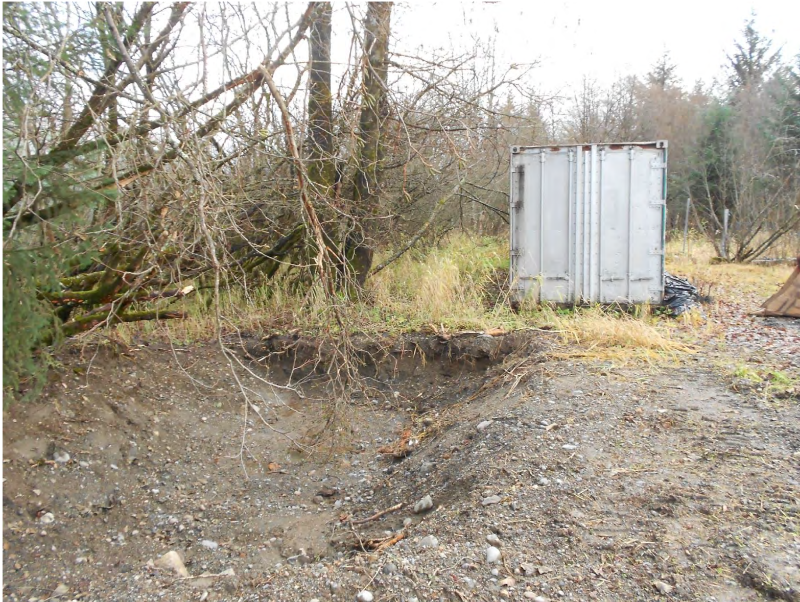
Figure 23. Close-up of the rain garden excavation. Photo taken November 2015.
