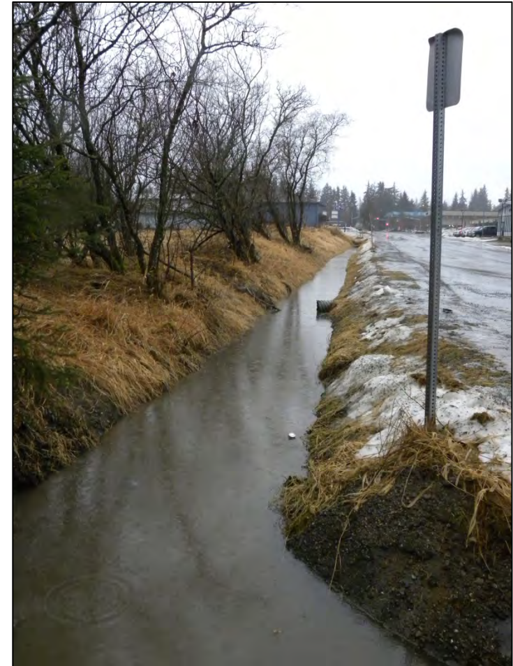
South Jordan Ave. ditch
