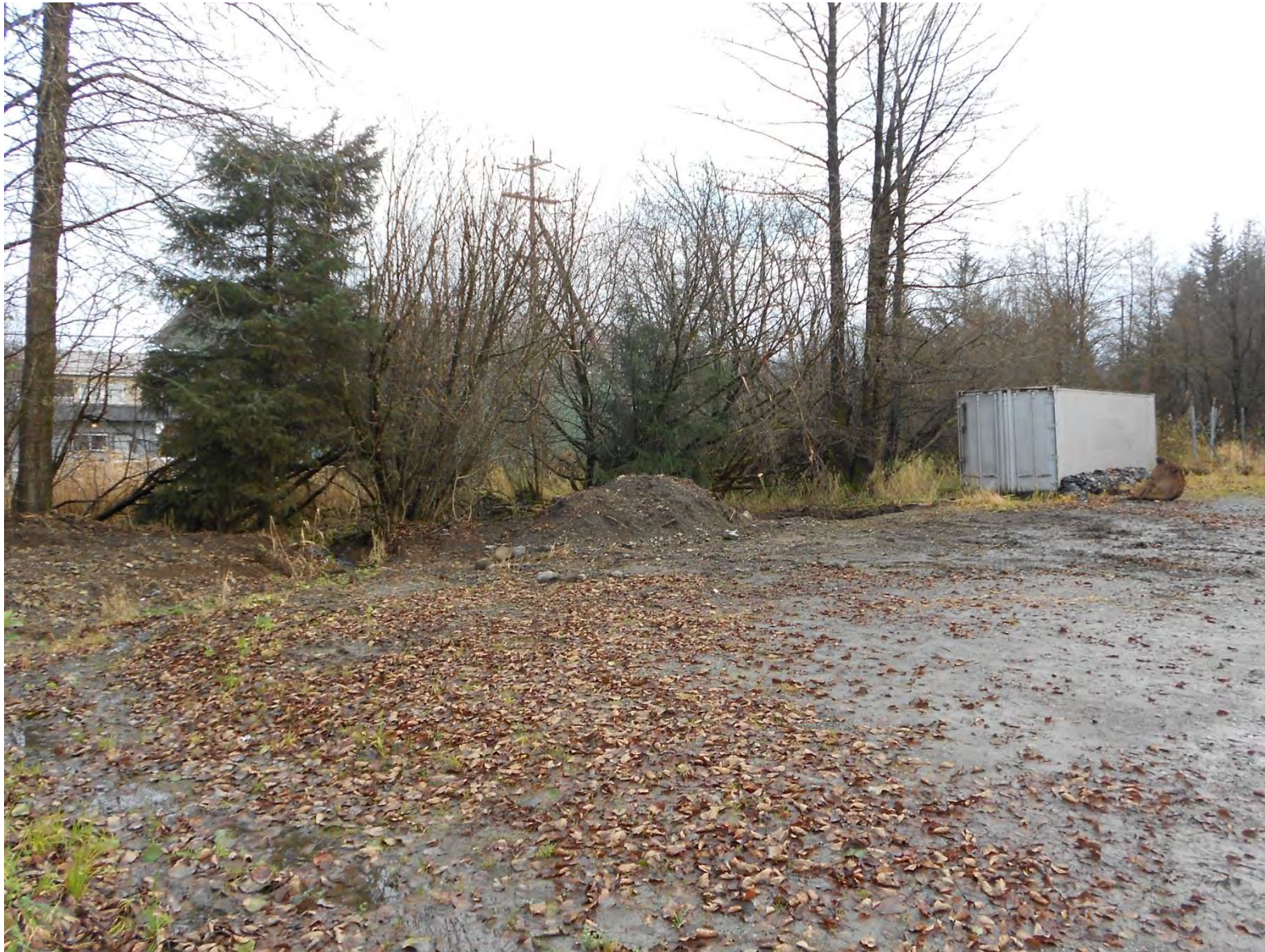
Figure 22. Start of rain garden excavation. Photo taken November 2015.
