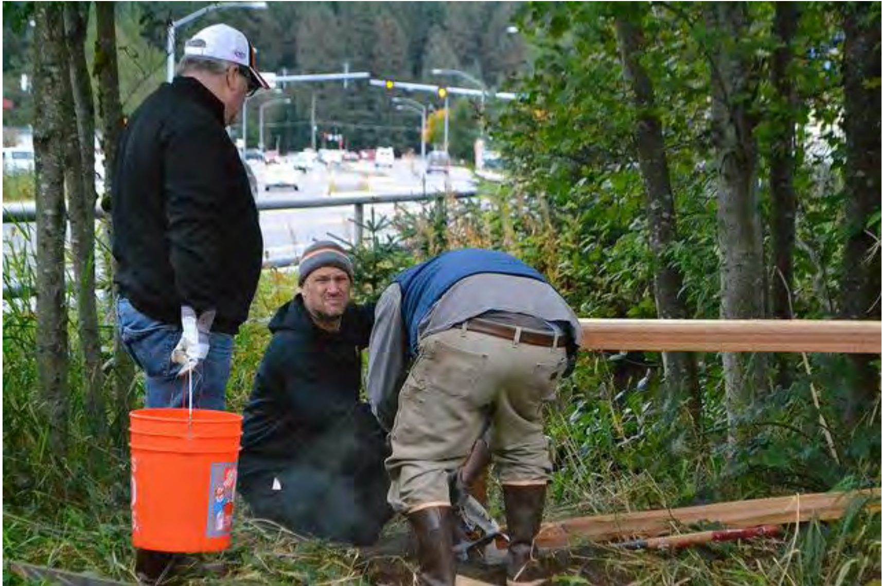
Figure 10. Installing the first length of fence. Photos taken September 2015.
