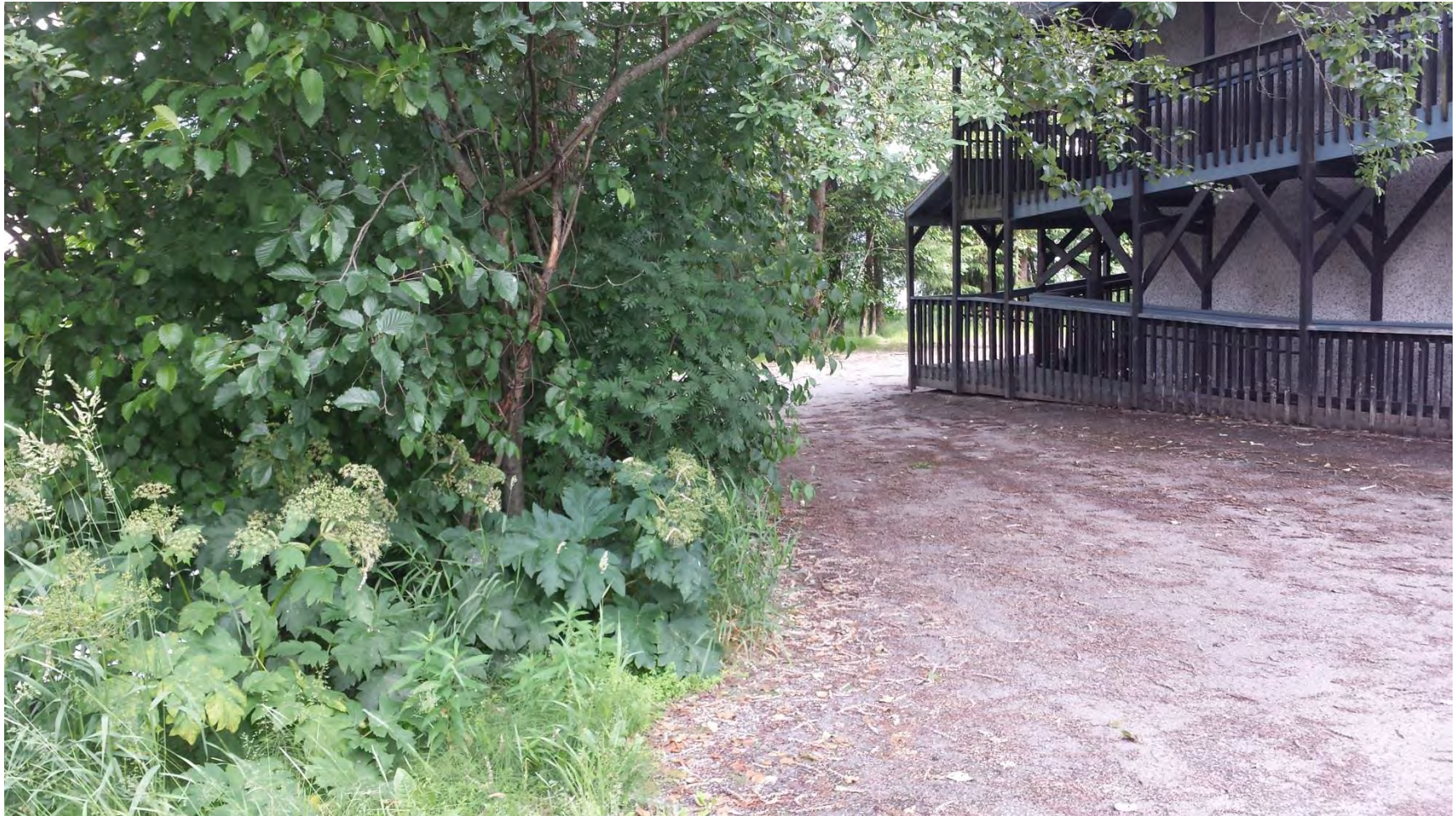
Figure 2. North side of the Edward K Thomas Building, looking east toward back parking lot. Photo taken June 2015.
