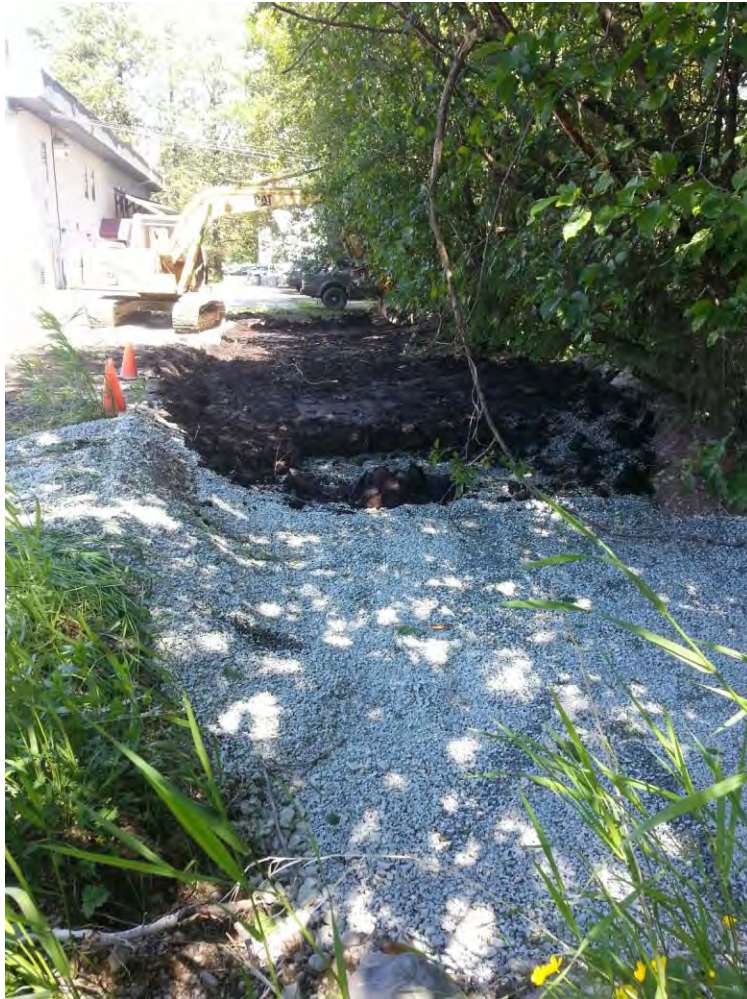
Figure 36. Another view of the drain rock and top soil in the rain garden, at various stages of placement. Photo on left taken by Dave Hanna, SOURCE, LLC., on June 9, 2016. Photo on right taken by JWP on June 11, 2016 prior to planting.
