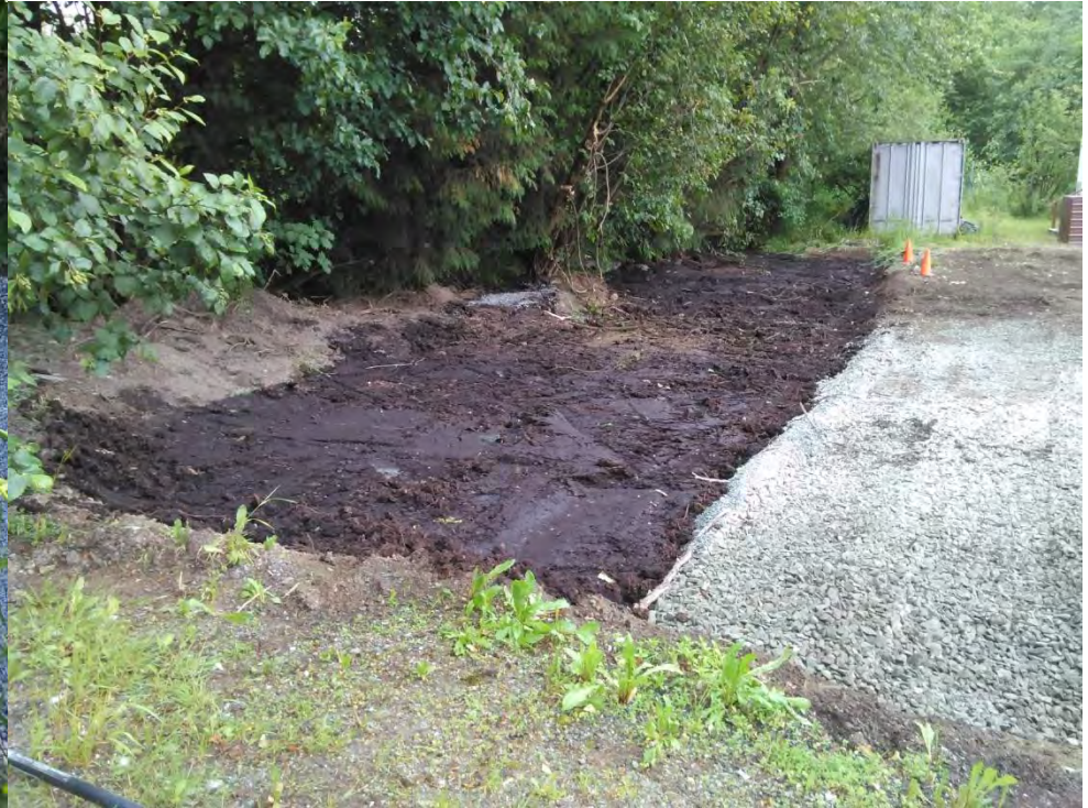
Figure 36. Another view of the drain rock and top soil in the rain garden, at various stages of placement. Photo on left taken by Dave Hanna, SOURCE, LLC., on June 9, 2016. Photo on right taken by JWP on June 11, 2016 prior to planting.
