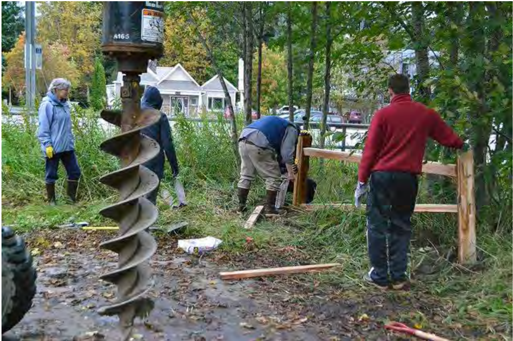
Figure 11. Installing the first length of fence. Photos taken September 2015.
