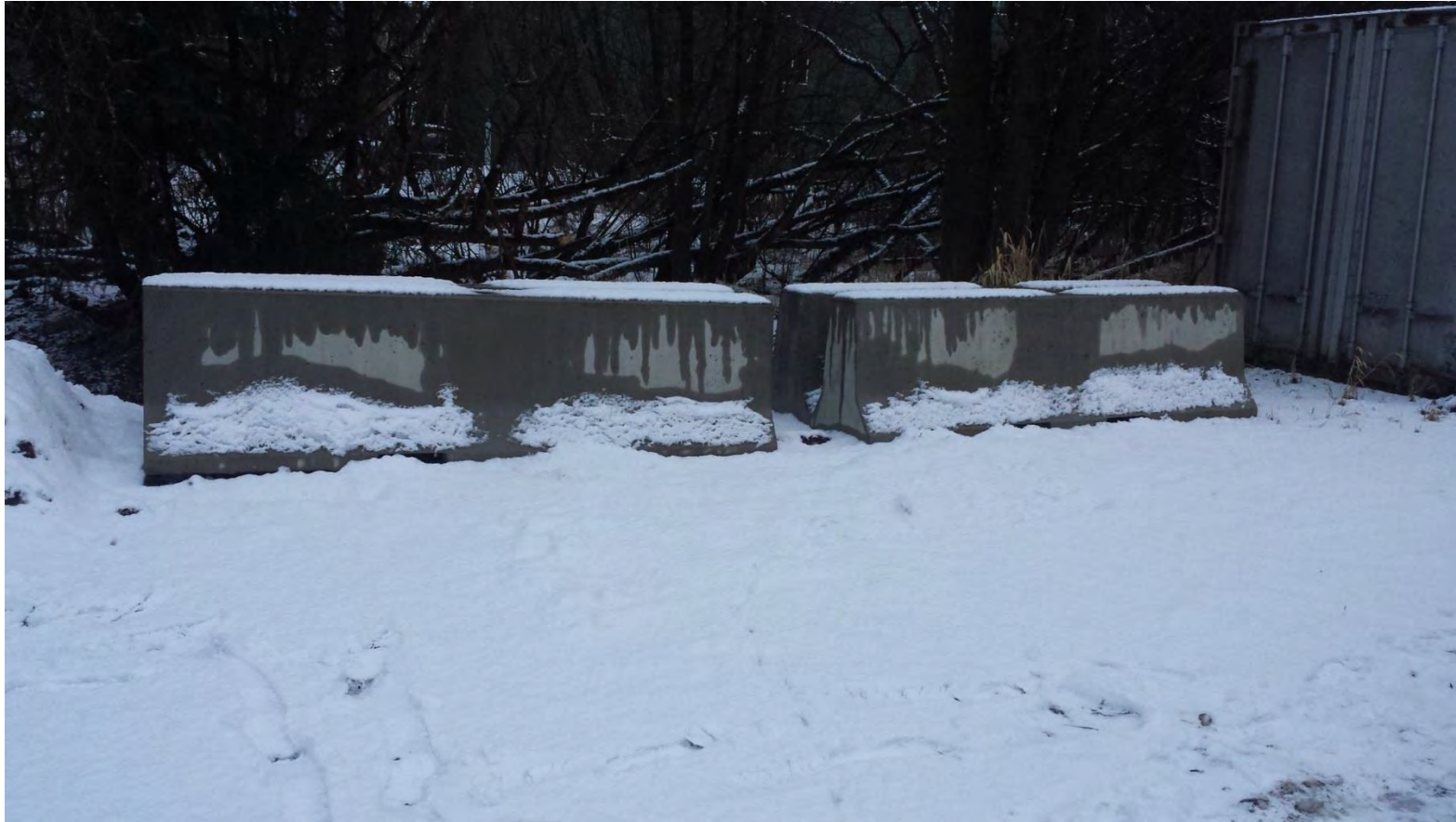
Figure 27. Concrete barriers protecting rain garden. Photo taken December 2015.
