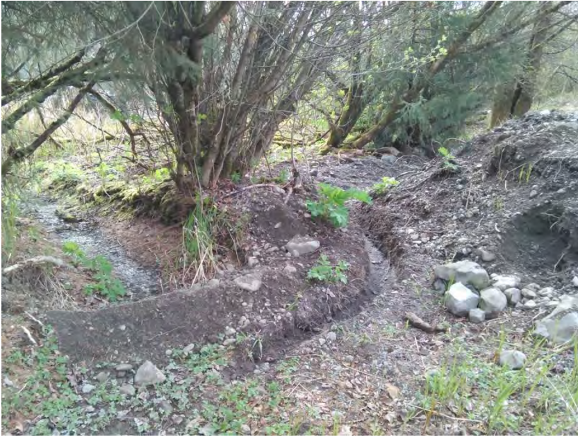
Figure 28. Diversion ditch to divert run off into the excavated hole that will eventually become the rain garden. Photo taken April 2016.
