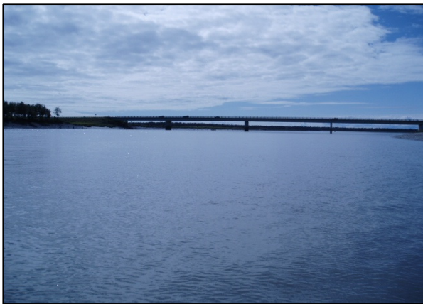
FIGURE 3: RM 5 ABOVE WARREN AMES BRIDGE
