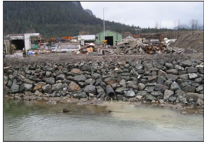
Figure 14: Turbid stormwater discharge into Lemon Creek from a failing oil-water separator at the (removed) Juneau ReadMix Bridge site, May 2007. Photo: S. Seifert.
