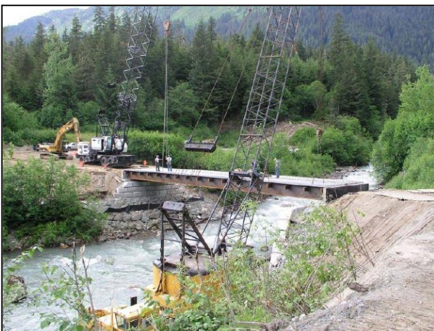
Figure 15: Construction of the CBJ Upper Lemon Creek Bridge (completed July 2007). Photo: Bob Millard, CBJ project manager, June 14, 2007.
