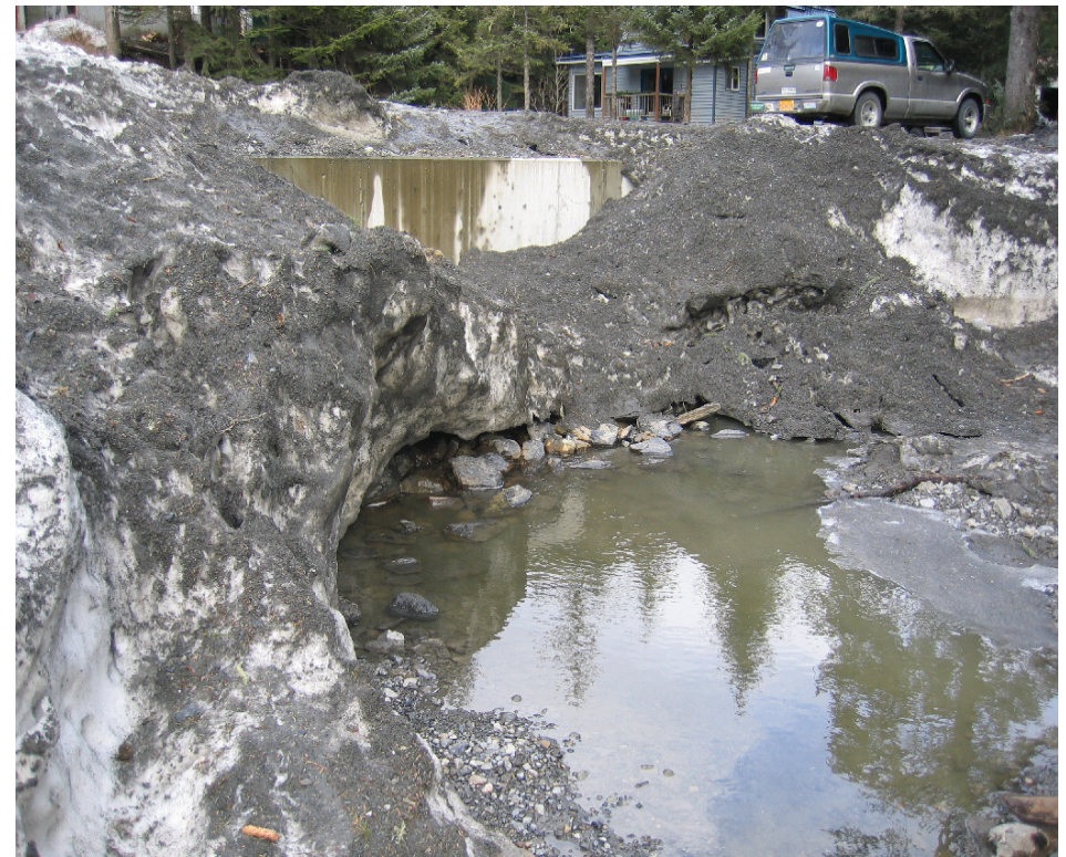
Street water run-off and sediments enter Eyak Lake through unfiltered culverts and from heavy precipitation events carrying gravel used in winter for road traction. Uncombusted fuel, leaking fluids from vehicles, and spills account for detectable levels of PAHs in Eyak Lake. This culvert site near Nirvana Park, Cordova, AK was also used as a snow dump during the 2006 - 2007 winter (photo taken in March, 2007).
