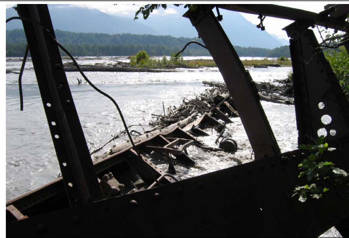
Another view looking at the railroad car section that shows how it provides some bank erosion protection from the Matanuska River. (7/16/04)
