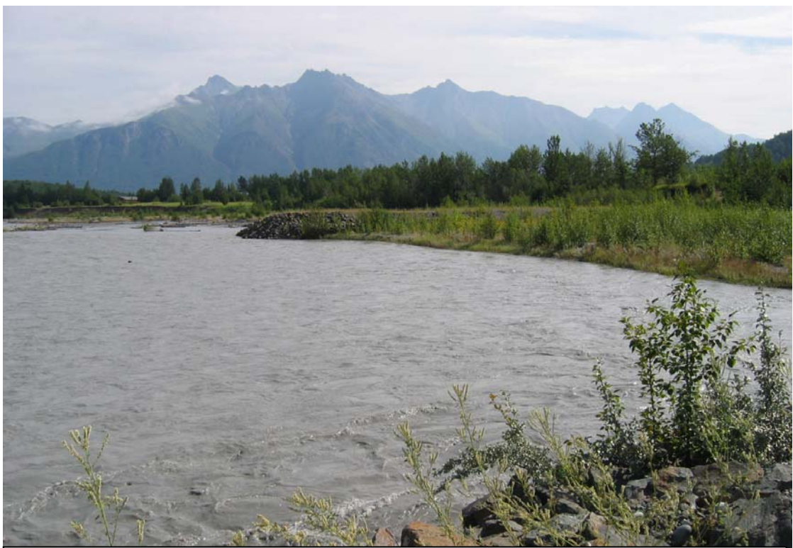
Matanuska River bank stabilization efforts in the Bodenbug Butte area. These large rock finger dikes were constructed in 1992 to prevent further bank erosion. (7/16/04)
