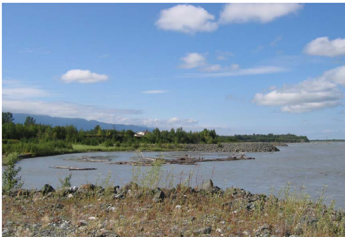
Looking downstream at additional rock finger dikes in the Bodenbug Butte area. Notice that some bank erosion has occurred between the two closest dikes. (7/16/04)
