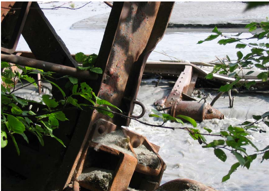
Additional rail car debris laying in a channel of the Matanuska River. (7/16/04)
