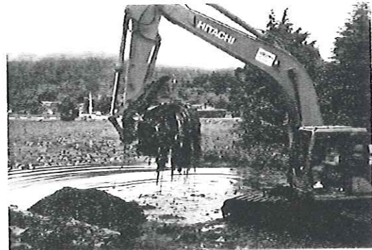
Vegetation and sediment removal, Swan Lake outlet channel, June 19, 2001
