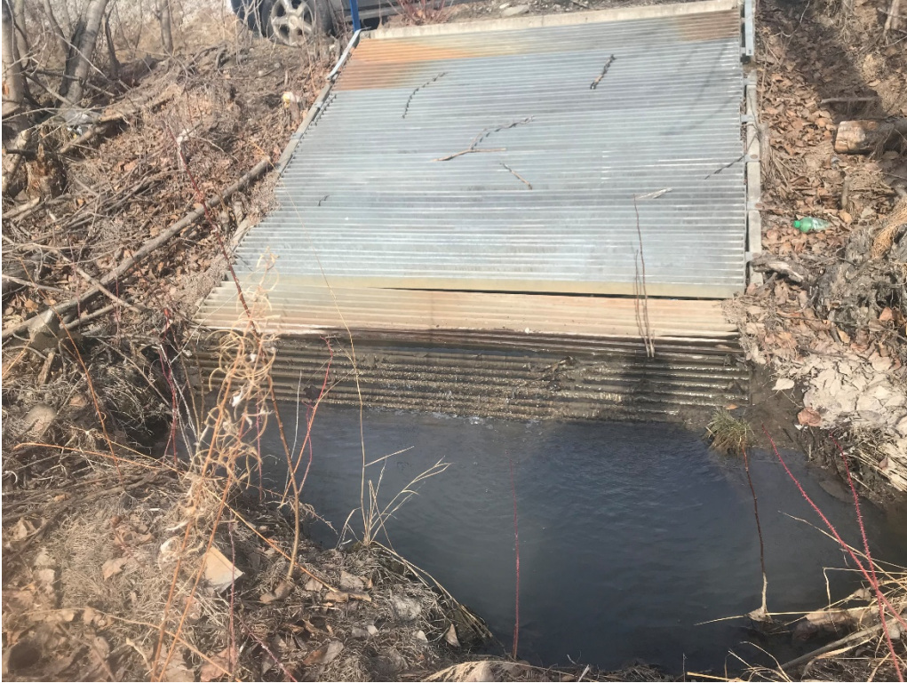
Photograph A7. Discharge from east outfall on 3/22/19.
