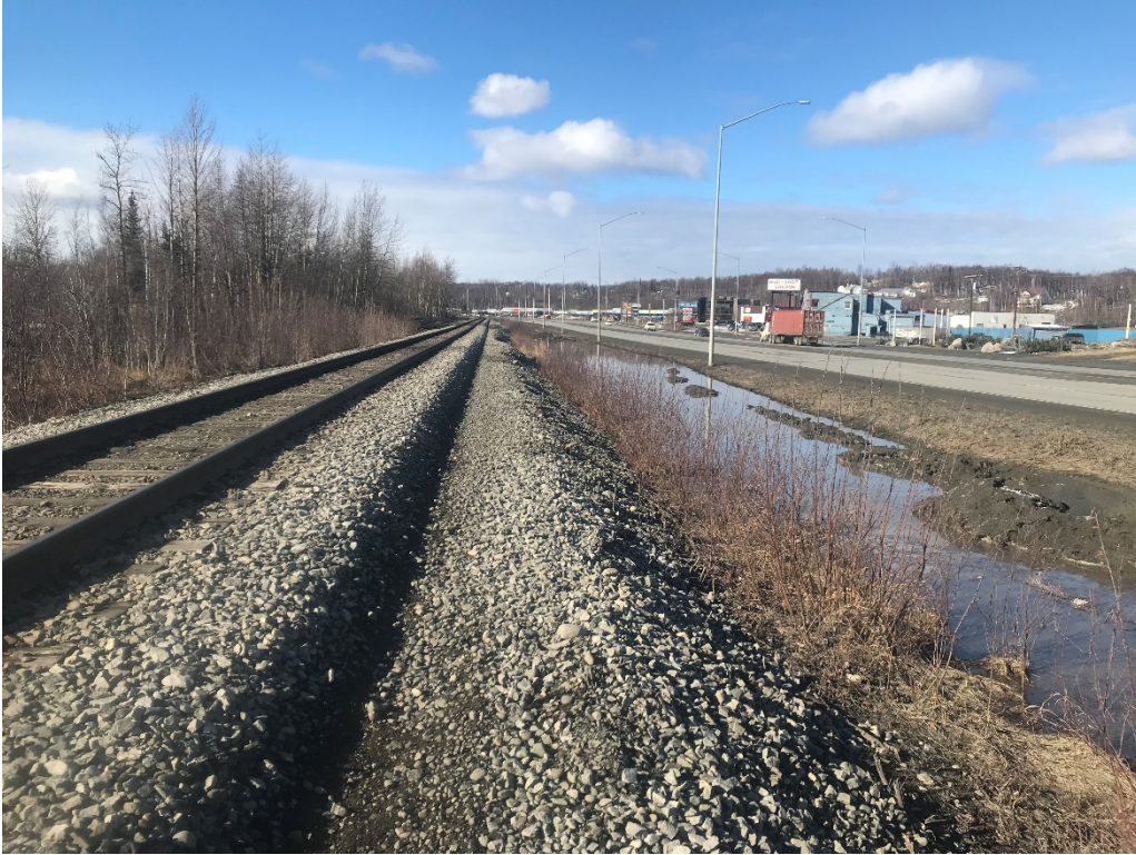
Photograph A5. Snow storage and runoff between the Parks Highway and the ARRC tracks near the east outfall. (3/19/19)
