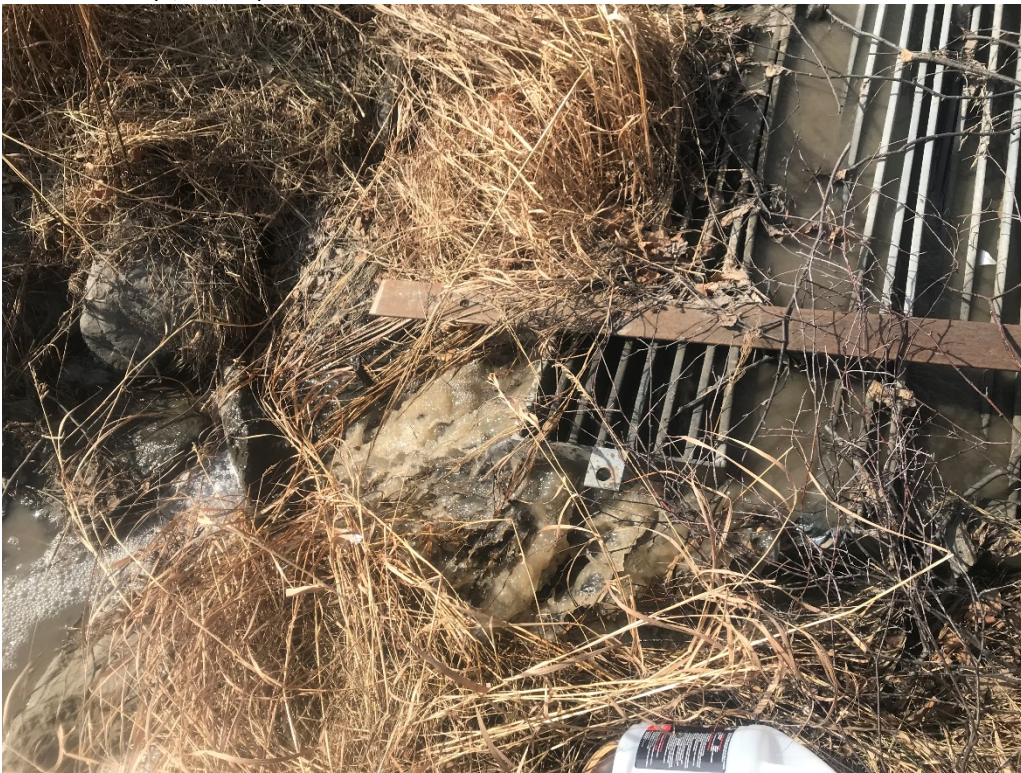
Photograph A6. Turbid runoff from west outfall on 3/22/19.
