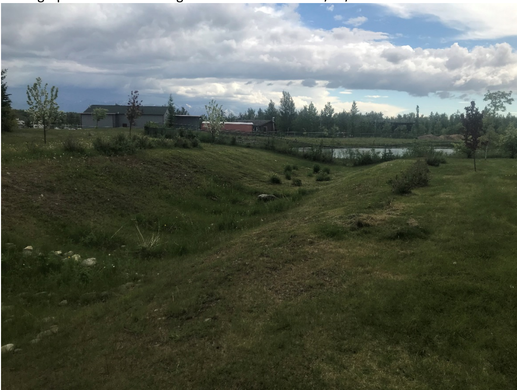
Photograph A9. Vegetated swale from Nelson Avenue to Iditapark Retention Pond. (6/3/19)
