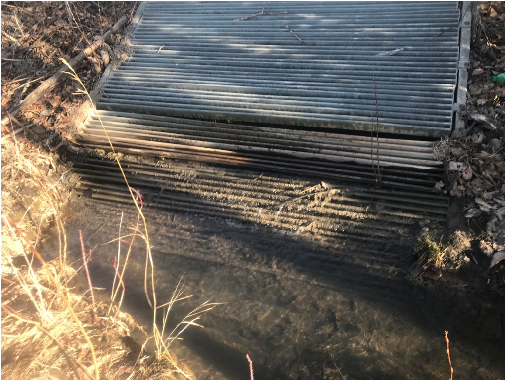
Photograph A8. Clear discharge from east outfall on 3/26/19.
