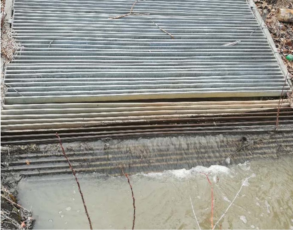
Photograph A3. East outfall. (3/18/19)
