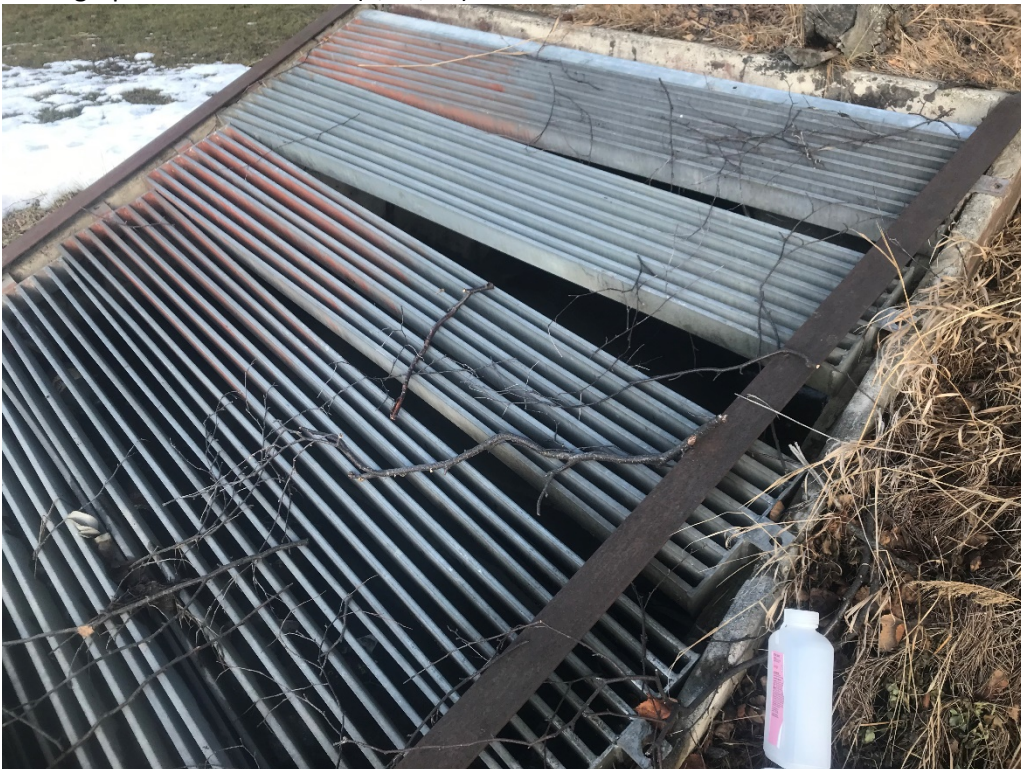
Photograph A2. West outfall. (3/19/19)
