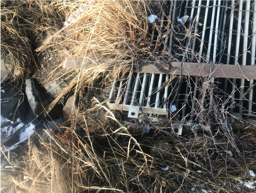
Photograph A1. West outfall. (3/19/19)
