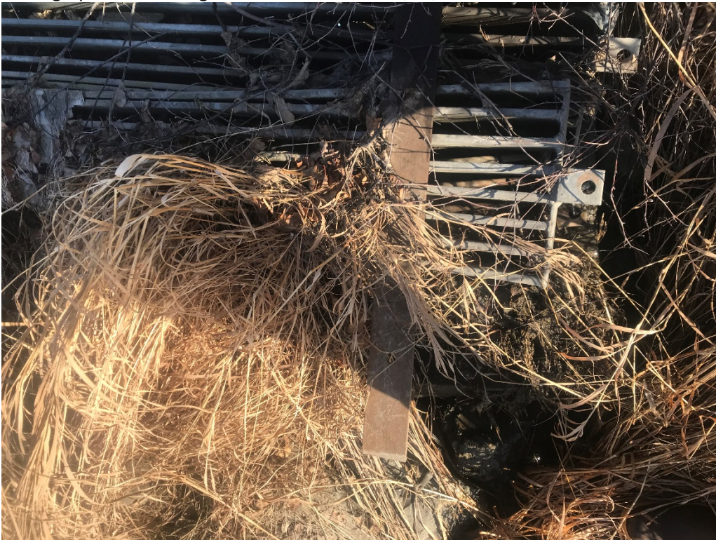
Photograph A7. No discharge from west outfall by 3/26/19.
