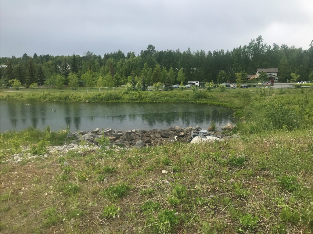
Photograph A10. Discharge outfall to Iditapark retention pond. (6/3/19)
