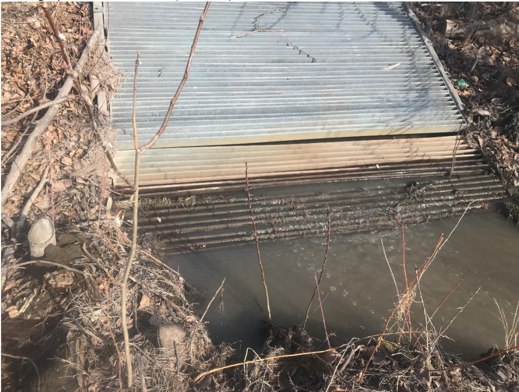
Photograph A3. Turbid discharge from east outfall. (3/19/19)
