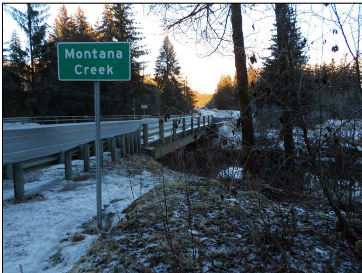
Figure 11. The Montana Creek Bridge located on Back Loop Road. Photo courtesy of Amy Sumner, JWP.
