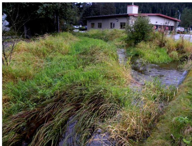
Figure 13. Reed canarygrass blocking one of the Jordan Creek Glacier Highway culverts during a high flow event. The culvert being blocked is in the center foreground of the photo, to the left of the culvert passing water.
