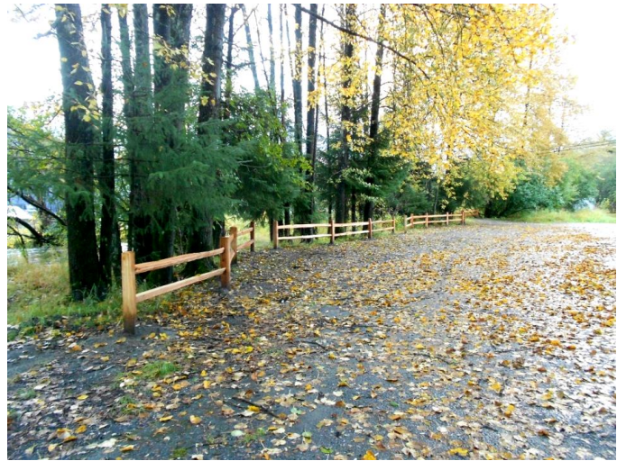
Figure 20. Successful riparian fencing installed on Jordan Creek at the Edward K. Thomas building owned by the Central Council of Tlingit and Haida.
