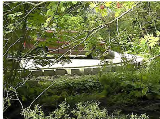
Figure 41. Successful streambank stabilization behind Race Realty. Photo from JWP Archives.
