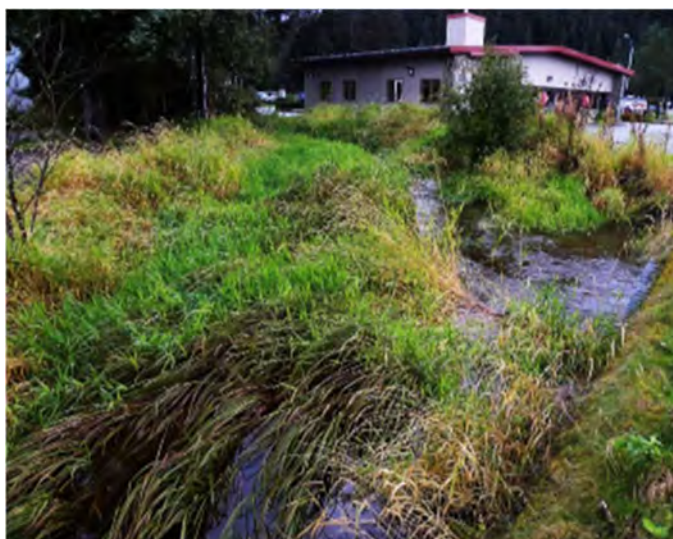
Figure 38. Reed canarygrass constricting the channel of Jordan Creek and blocking flow from passing through one of the Glacier Highway culverts.
