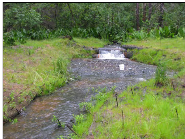
Figure 40. The East Valley Reservoir tributary before (above) and after (below) restoration. Photos from JWP's archives.
