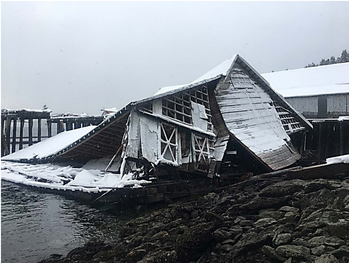
Photo of collapsed building containing bladder Taken March 10, 2018 Photo credit: Global Diving and Salvage Inc.
