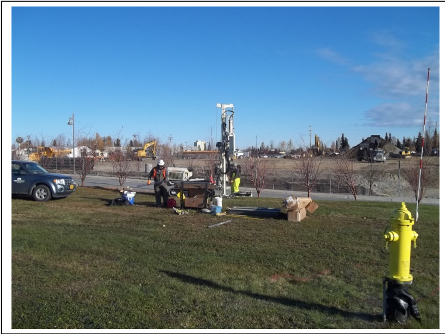
Photo 5: Advancing Boring B9; looking northeast. (October 8, 2014)
