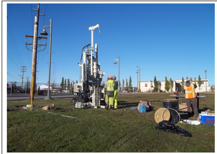
Photo 2: Advancing Boring B6; looking northwest. (October 7, 2014)
