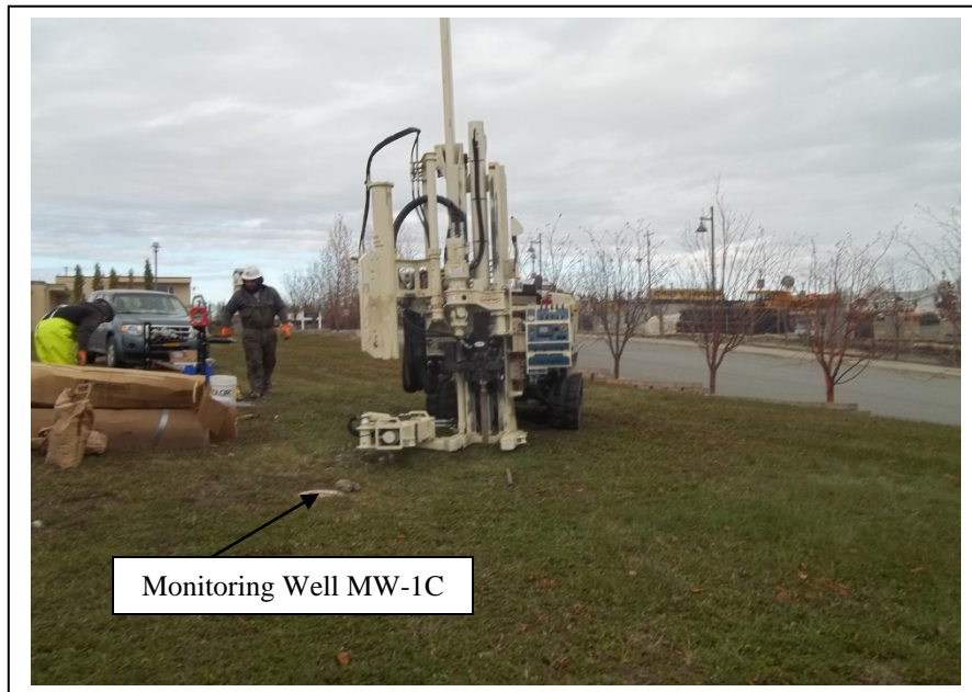
Photo 6: Advancing Boring B10; looking north. (October 8, 2014)
