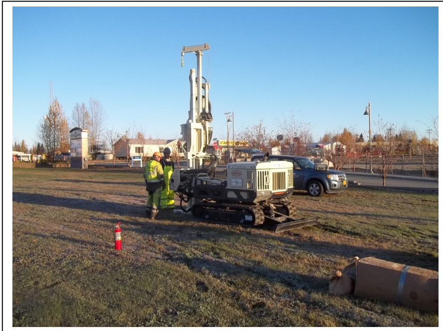
Photo 1: Advancing Boring B5; looking north. (October 7, 2014)
