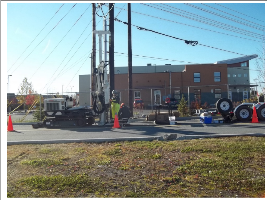
Photo 3: Advancing Boring B7; looking west/southwest. (October 7, 2014)
