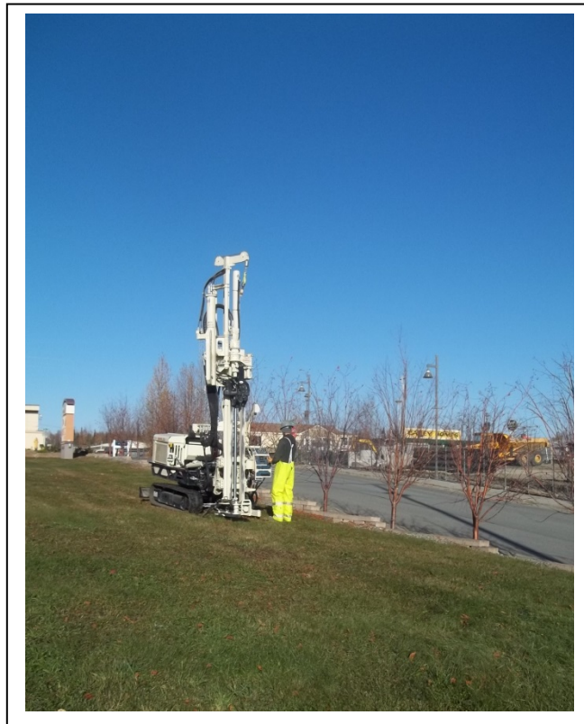
Photo 8: Advancing Boring B12; looking north. (October 9, 2014)
