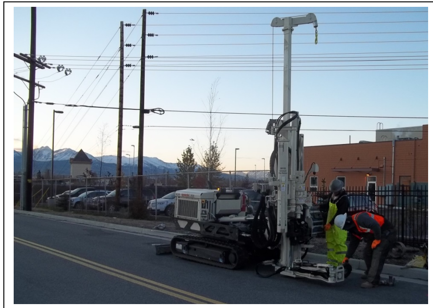
Photo 4: Advancing Boring B8; looking south. (October 8, 2014)
