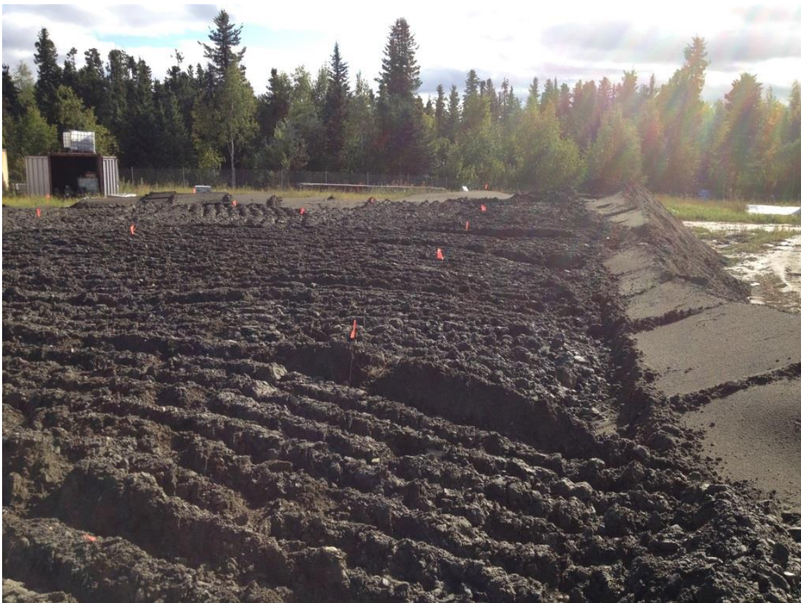
10) Landspread contaminated soil in area north of previously (2013) landspread soil, separated by soil berm. August 29, 2014.
