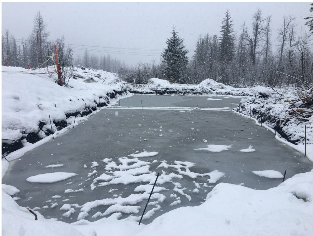
Excavated area of the spill site, 3/19/2018 (Photo by ADEC)
