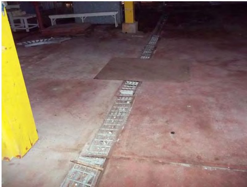
Photo 14: Strip drains in cleaning room. (February 3, 2014)
