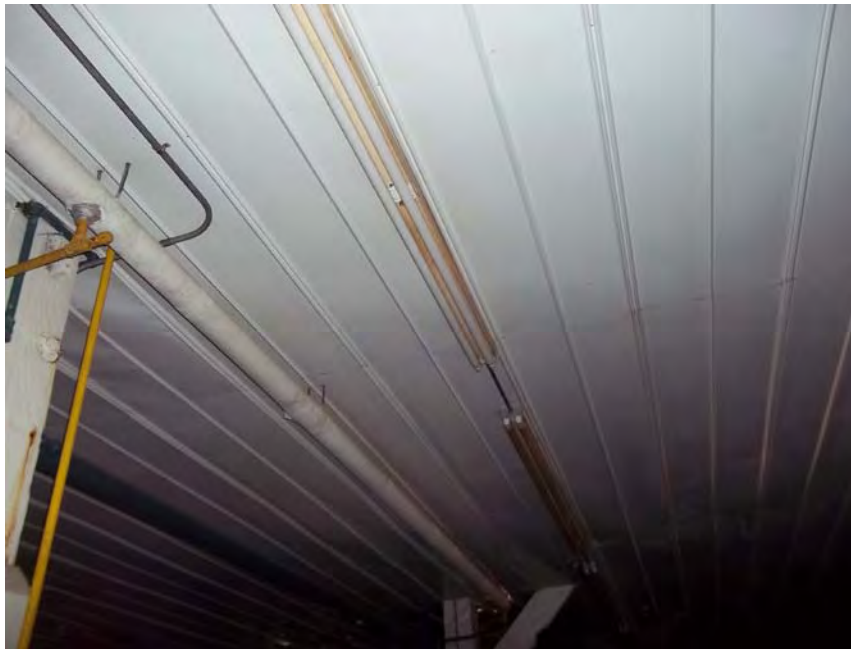
Photo 21: Presumed PCB-containing lighting in cleaning room. (February 3, 2014)
