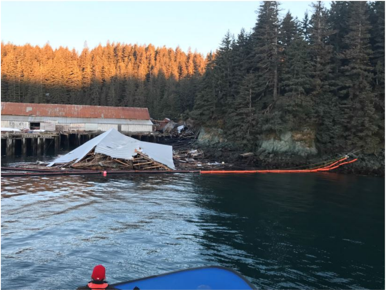
Photo of collapsed building containing bladder Taken March 21, 2018 Photo credit: Global Diving and Salvage Inc.
