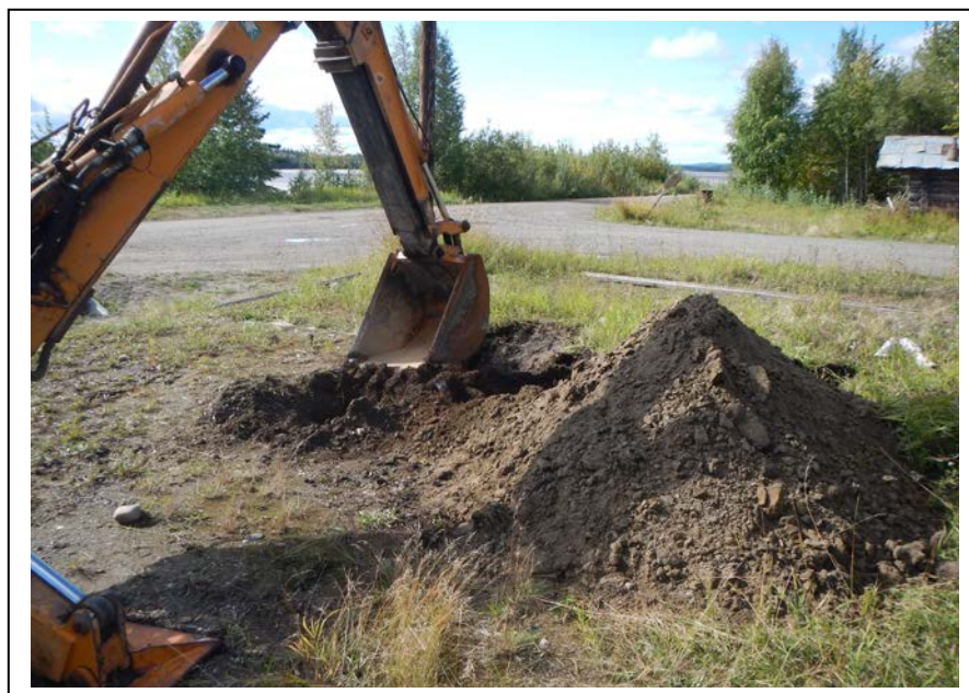
Photo 8: The excavation of Test Pit 1. Front Street (left), Koyukuk Street (right), and the Yukon River are visible in the background; facing southwest. (August 29, 2014)
