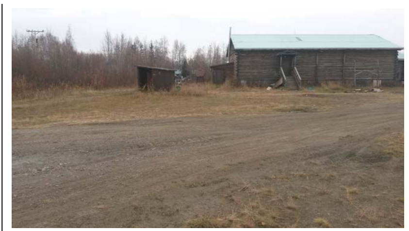
Photo 3: An informal roadway runs northwest-southeast across the Property, Tanana Community Hall in the background; facing east. (September 30, 2014)
