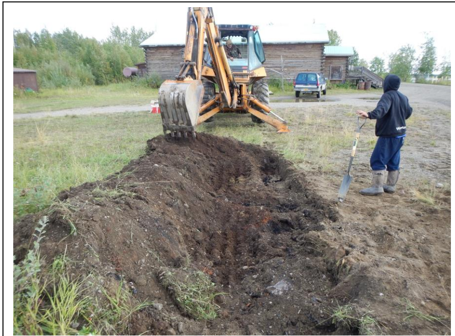
Photo 11: Excavating the Test Trench in the southern portion of the Property. Tanana Community Hall visible in background; facing east. (August 29, 2014)
