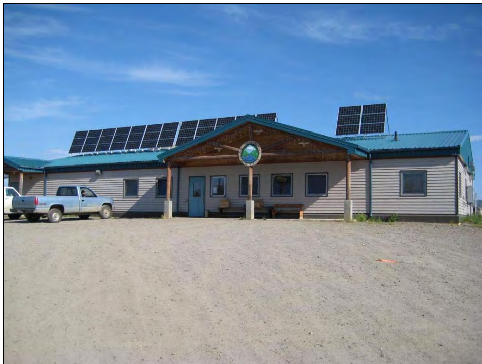
Photograph 4: The new water treatment and laundry facility.
