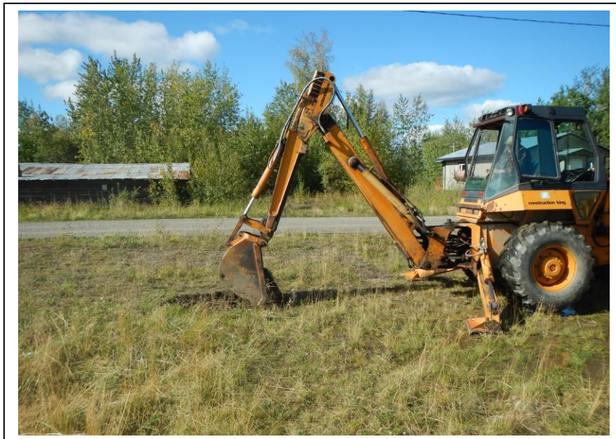
Photo 12: Excavation of Test Pit 2, in the northwestern quadrant of the Property. (August 29, 2014)
