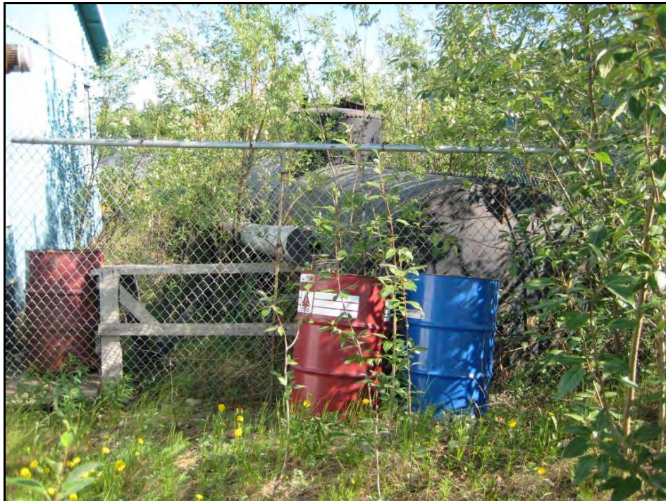
Photograph 20: 10,000 gallon train-car fuel tank used for heating the Former Washeteria site of environmental concern.
