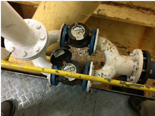
Photo 13: WW flow meters vessels were estimating volume, even when a meter was present and some meters were disconnected, making it difficult to quantify actual volumes discharged.
