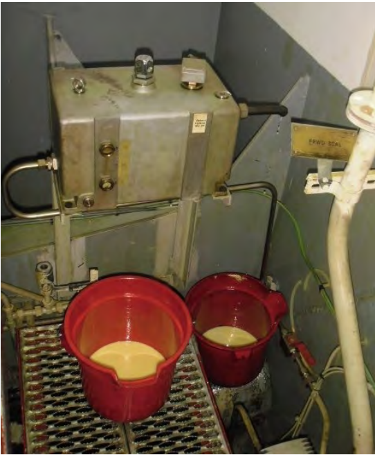
Photo 9: Example of leak potential into bilge
