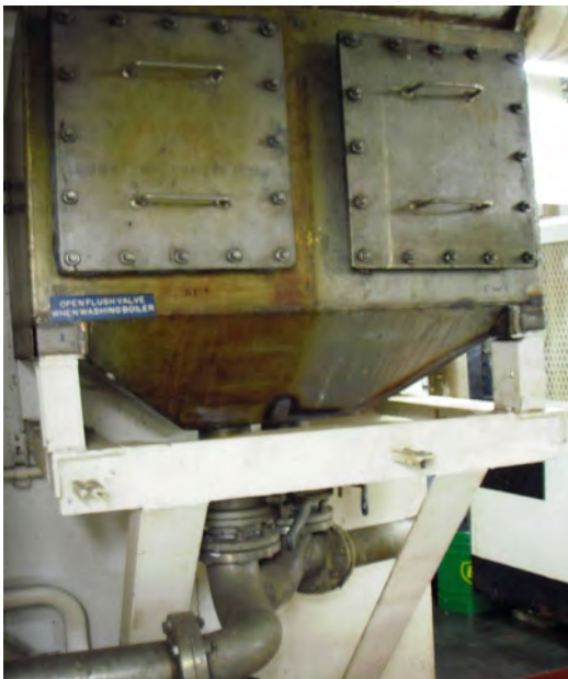
Photo 7: Boiler drain, soot trap
