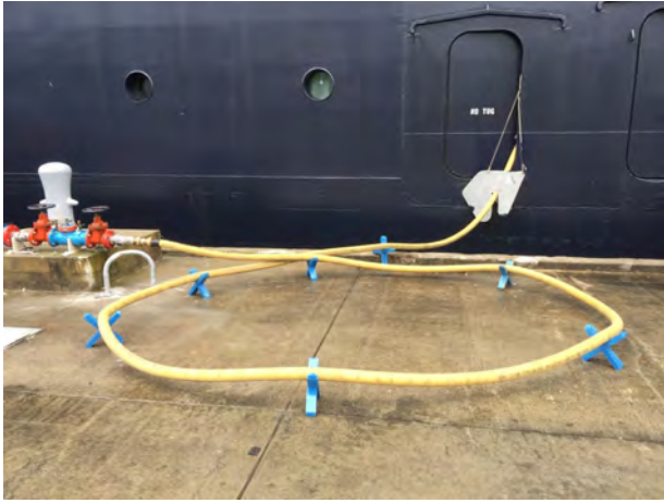
Photo 47: Elevated Potable water hose
