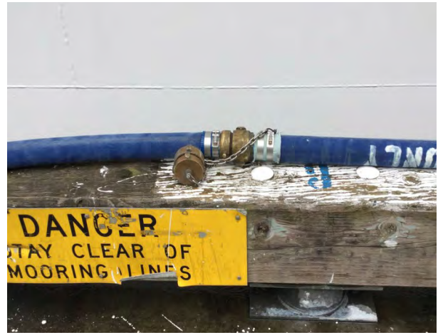
Photo 48: Potable Water hose & connection- Not 'free of the ground'
