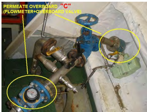
Photo 12: Overboard valve, flow meter, and Sample port
