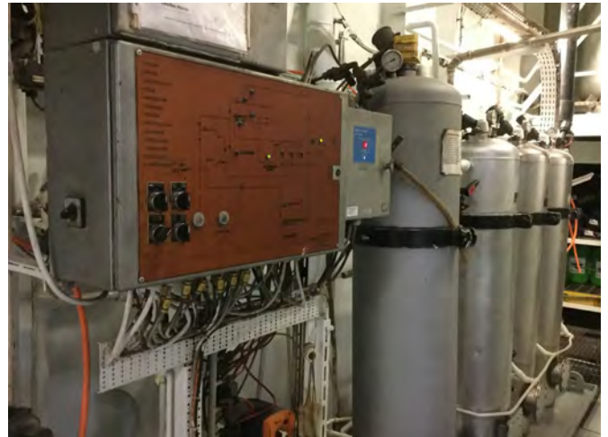
Photo 59: MarineFloc OWS Control panel
