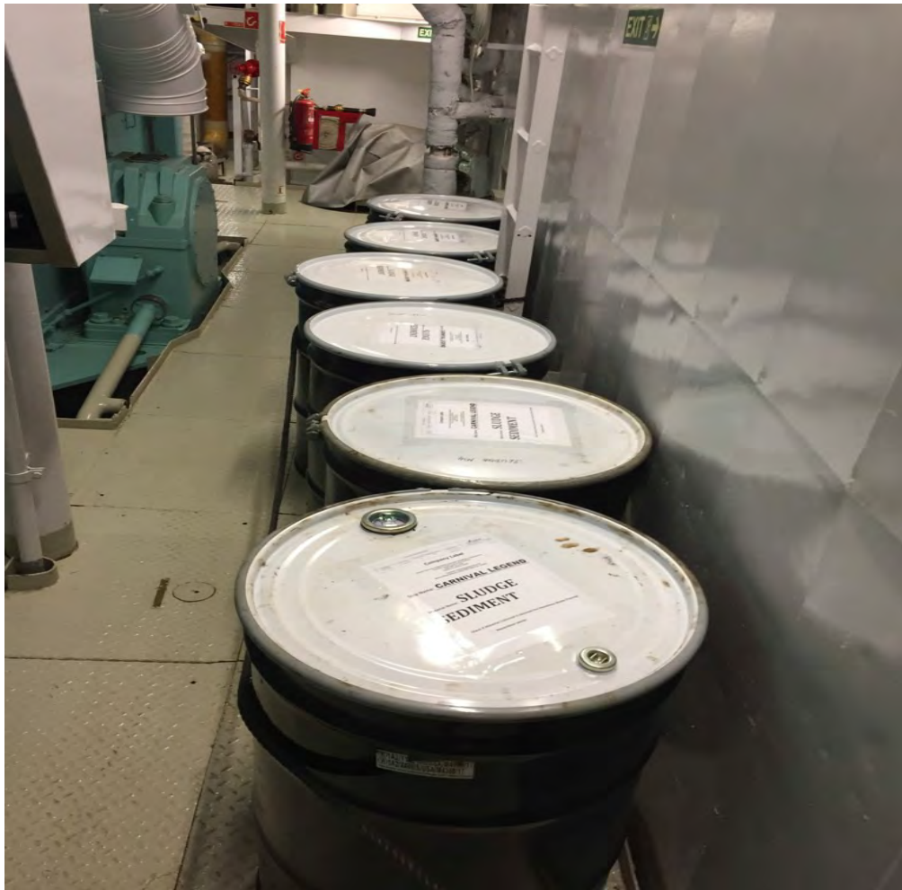
Photo 62: Oil Sludge Drums, stored for offload
