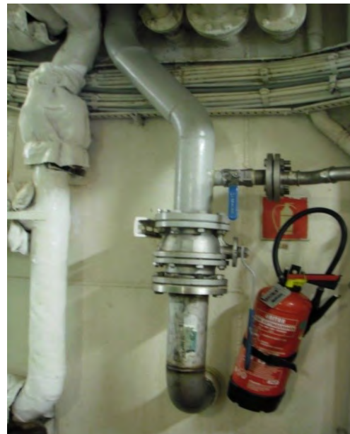
Photo 8: Boiler drain line
