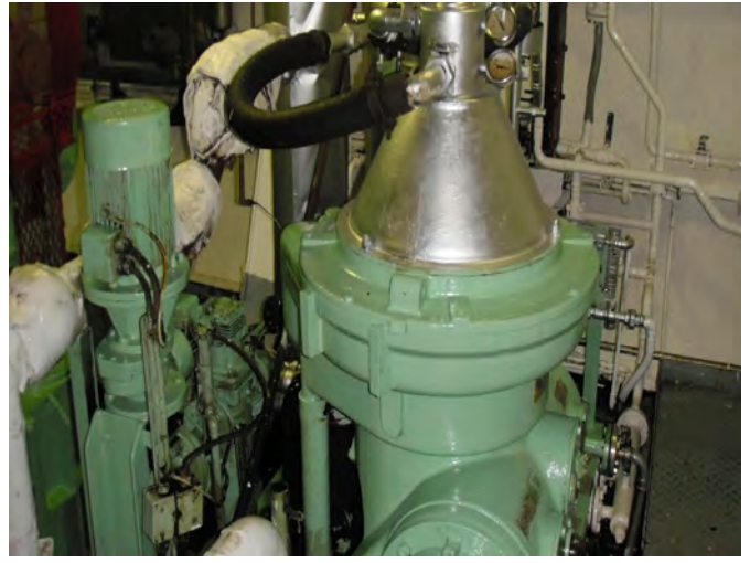
Photo 57: OWS separator/sludge treatment (dynamic) "concentrator"
