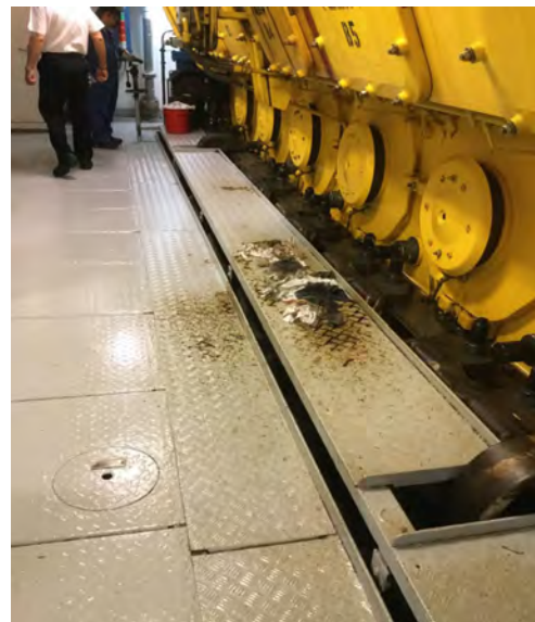
Photo 52: Internal oil leak, main engine
