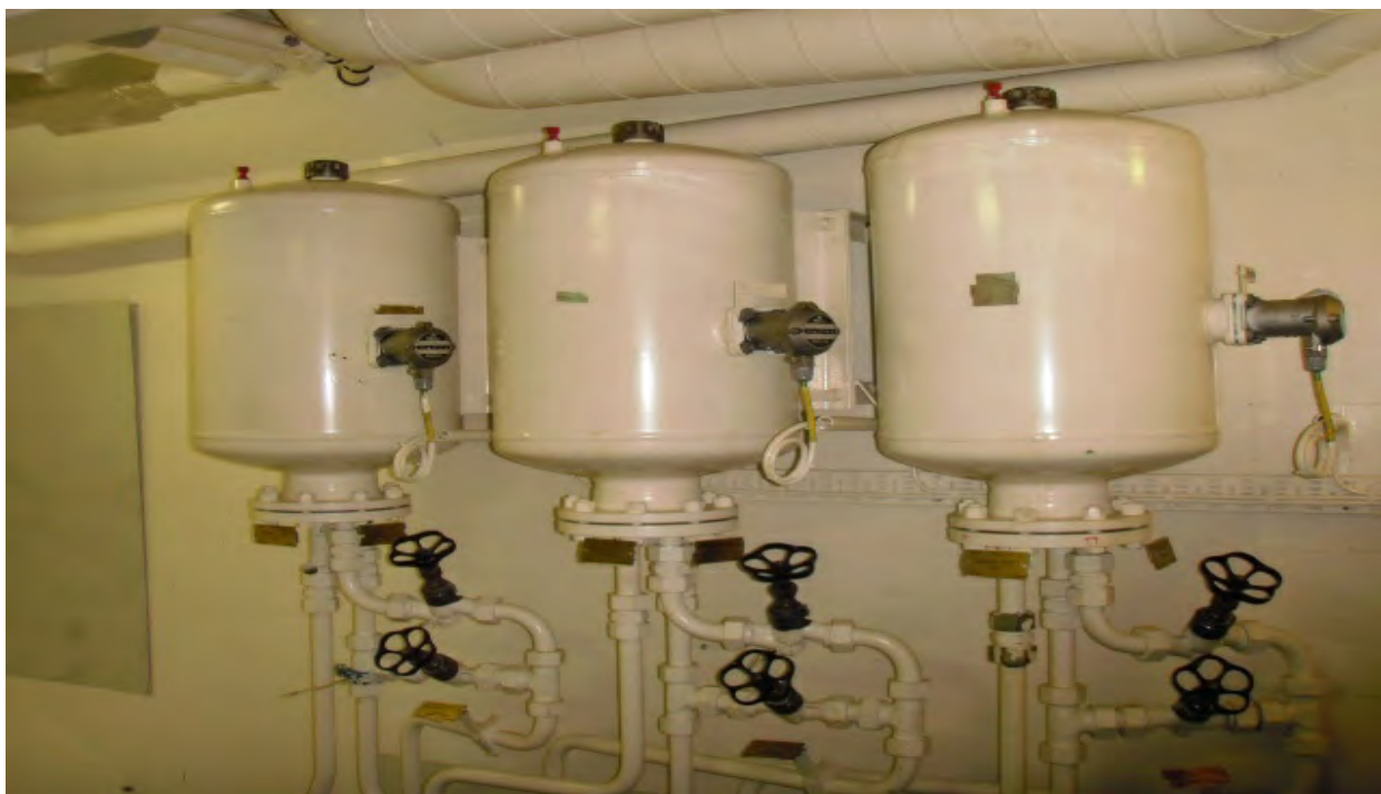
Photo 60: Oil to Sea gravity tanks
