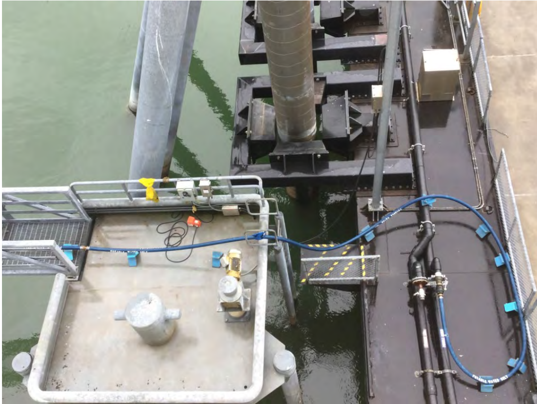
Photo 49: Water connection at dock
