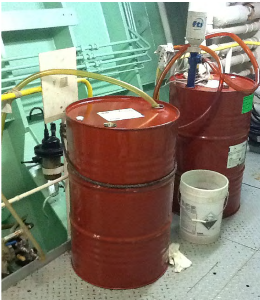
Photo 65: Temporary Oil filtration or Pumping system
