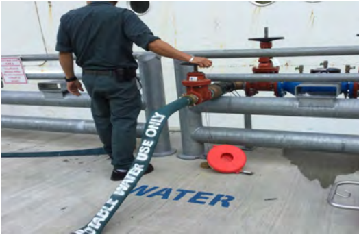
Photo 46: Potable Water Connection
