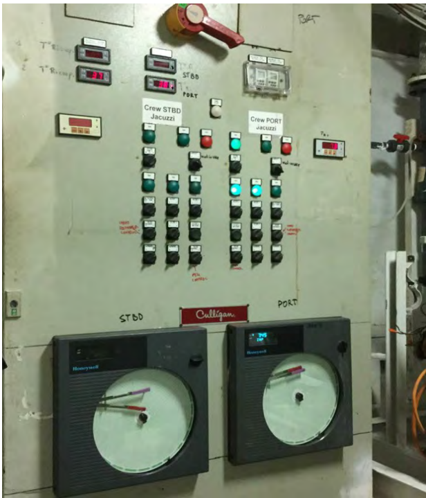
Photo 44: Pool Chemistry & Maintenance Room
