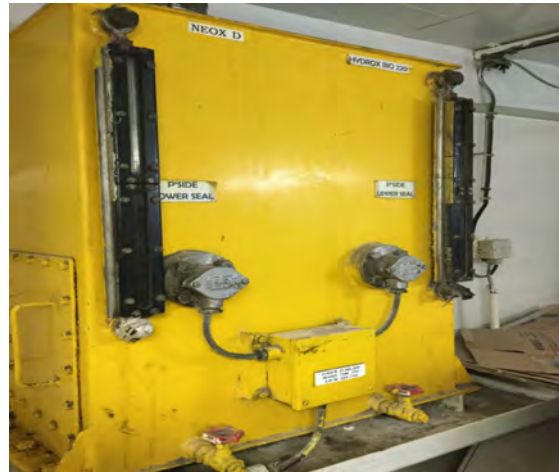
Photo 64: AZIPOD interface to sea head tanks & outer stern tube seals
