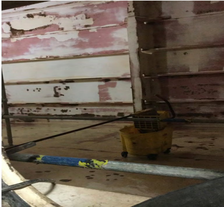
Photo 43: Safety 4, potential tripping hazard
