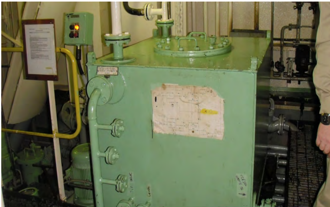
Photo 55: Concentrated Sludge Tank
