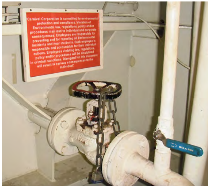
Photo 16: Closed discharge valve
