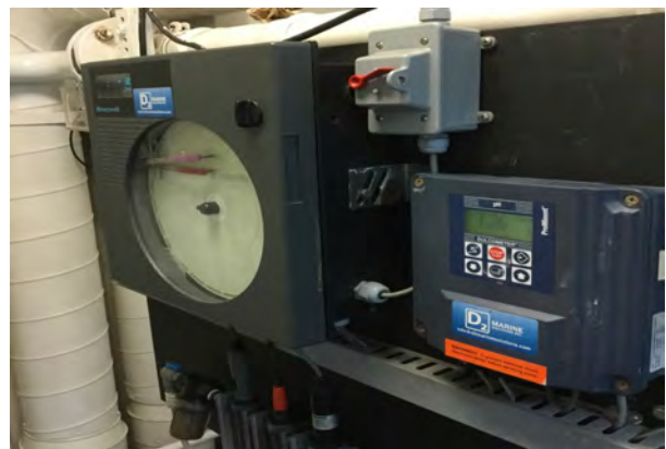
Photo 50: Chart Recorder for pH & Chlorination
