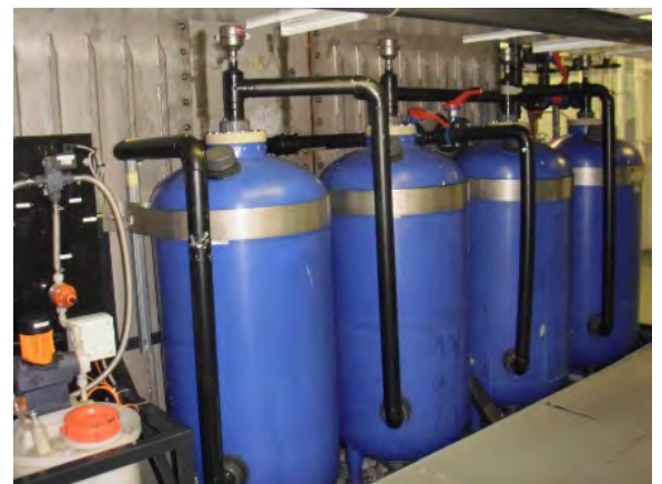
Regatta Ion Exchange tanks
