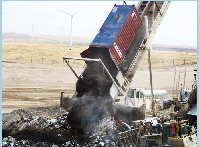
Offloading contaminated soil at Waste Management's Columbia Ridge Landfill, Arlington, Oregon
