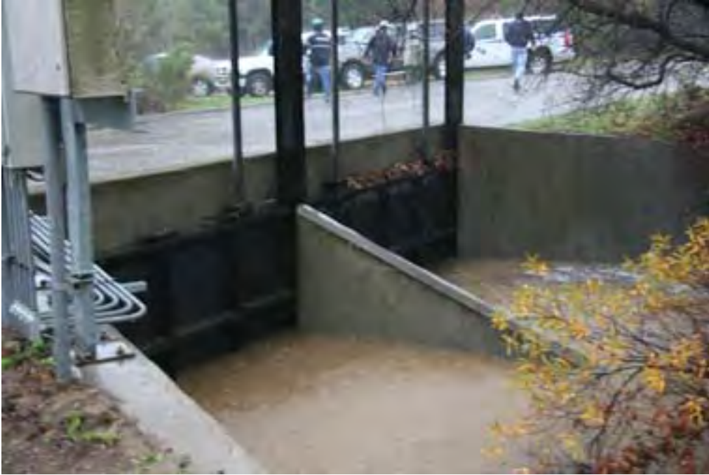
Weir gates on Corral Creek that attempted to contain contaminated water
