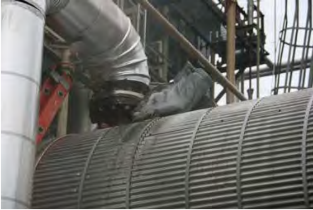
Location of failed flange gasket that caused leak
