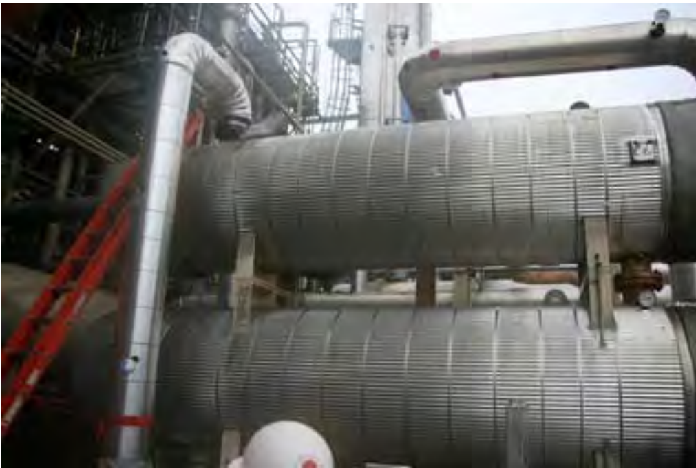
Gas processing exchanger units
