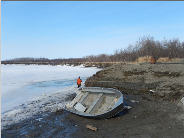
Figure 16. Akiachak - Riverbank Erosion 2013
