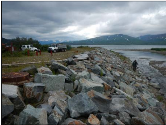
Figure 29. Chignik Lagoon - Revetment 2012
