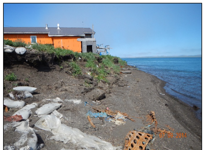
Figure 25. Kivalina - Shoreline Erosion 2014
