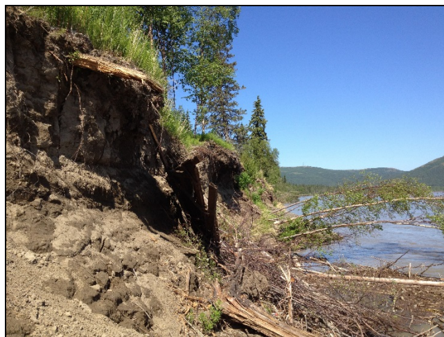
Figure 18. Lower Kalskag - Riverbank Erosion 2012
