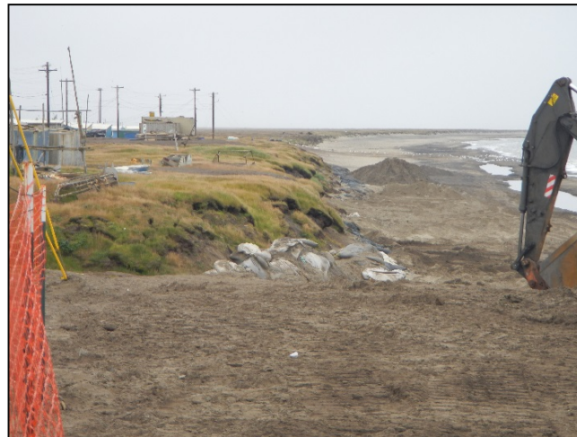
Figure 23. Wainwright - Shoreline Erosion and Riprap Installation 2013
