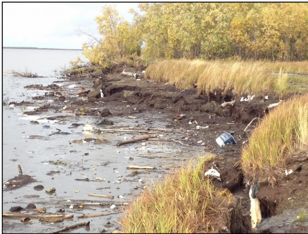
Figure 21. Mountain Village - Riverbank Erosion 2012
