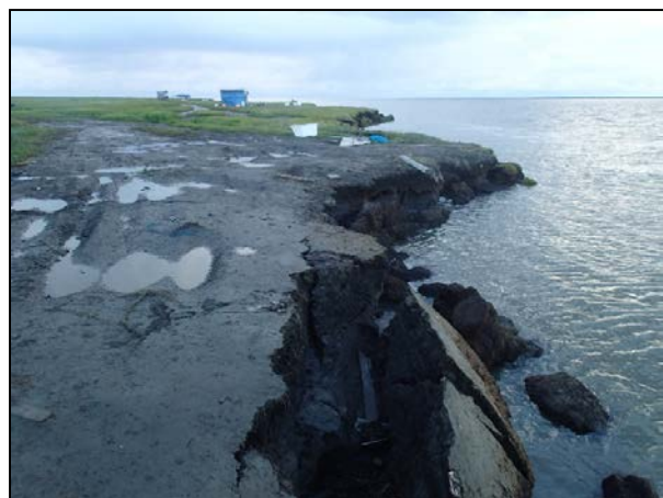
Figure 1. Nunam Iqua - Shoreline Erosion 2014
