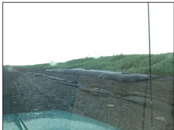
Figure 32. Nelson Lagoon - Geotube Erosion Mitigation 2013
