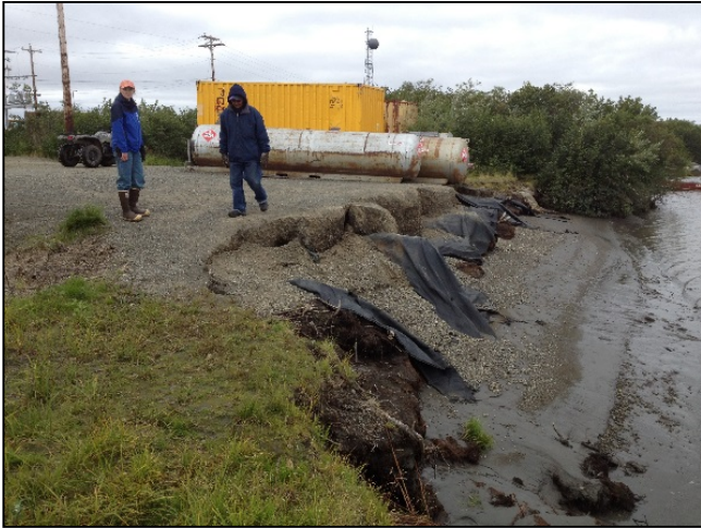
Figure 14. Tuntutuliak - Riverbank Erosion 2012
