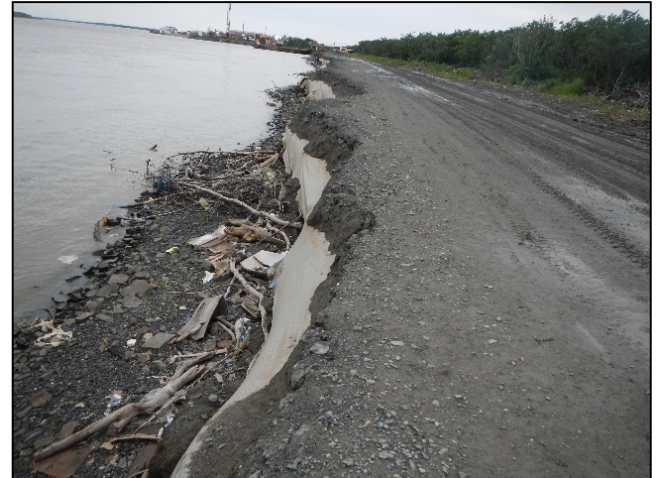
Figure 22. Emmonak - Riverbank Erosion 2014
