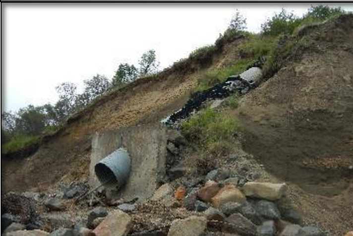
Water Outfall in Bluff (ADEC 2013)
