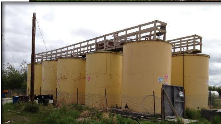
School Tank Farm (ADEC 2013)
