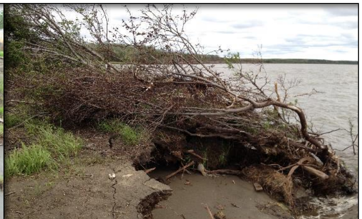
Kuskokwim River Erosion (ADEC 2013)
