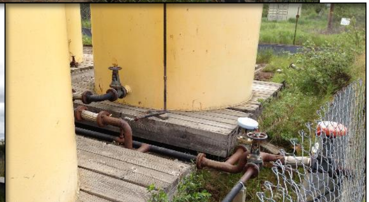
Fuel Lines and Timber Supports (ADEC 2013)
