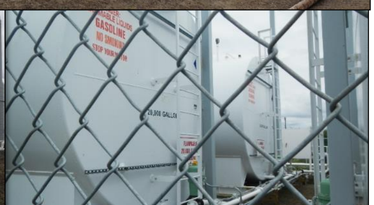
Corporation Tank Farm (ADEC 2013)
