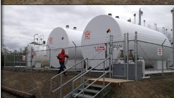
Corporation Tank Farm (ADEC 2013)
