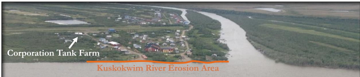
Aerial Photo Looking West (ADEC 2013)
