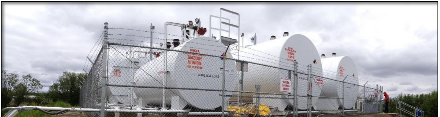
Corporation Tank Farm (ADEC 2013)
