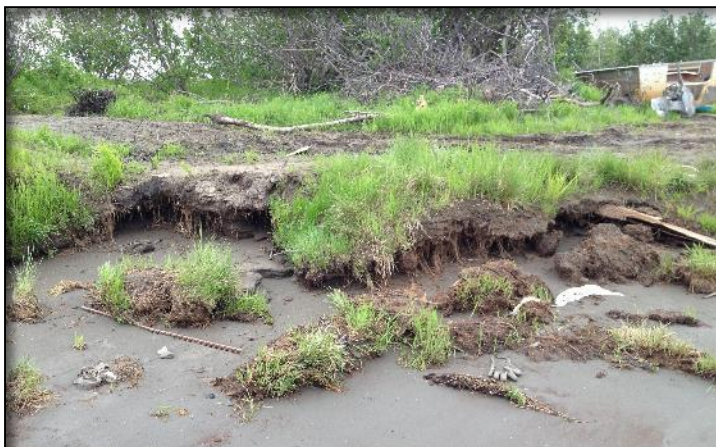
Kuskokwim River Erosion (ADEC 2013)
