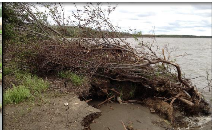
Kuskokwim River Erosion (ADEC 2013)
