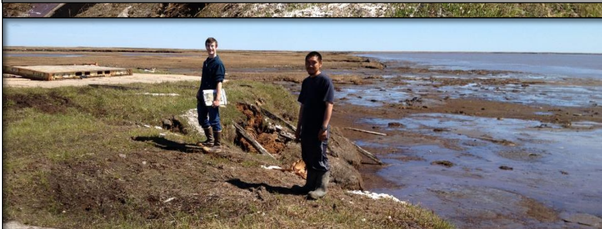
Ninglick River Erosion (ADEC 2013)
