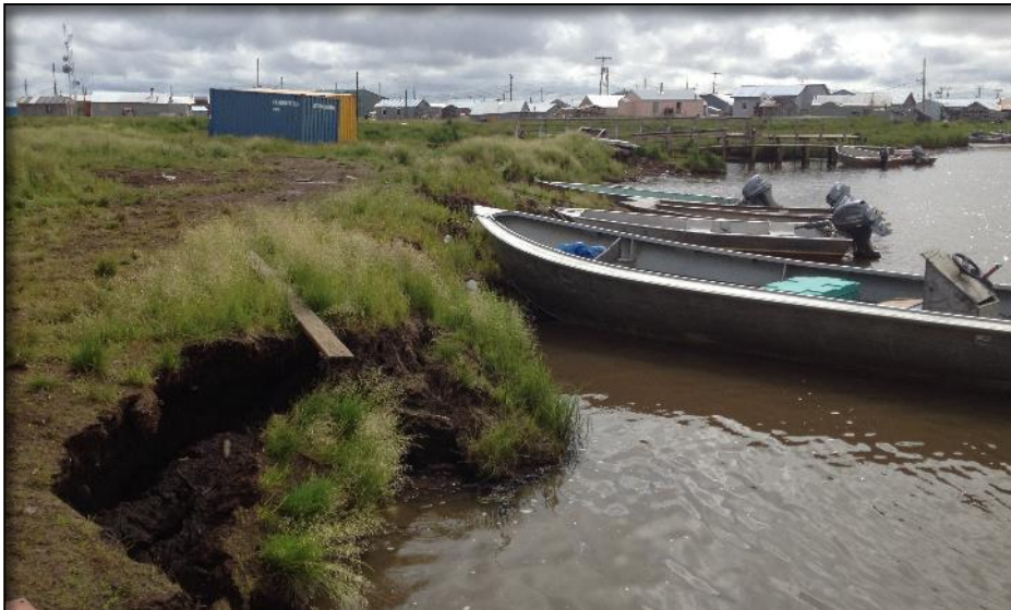
North Fork Johnson River, south bank erosion (ADEC 2014)
