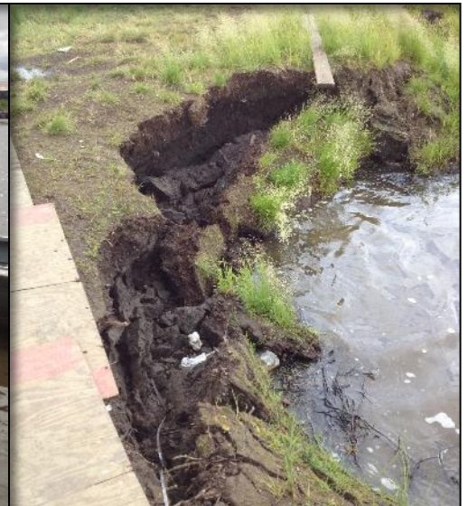
Eroding Riverbank (ADEC 2014)
