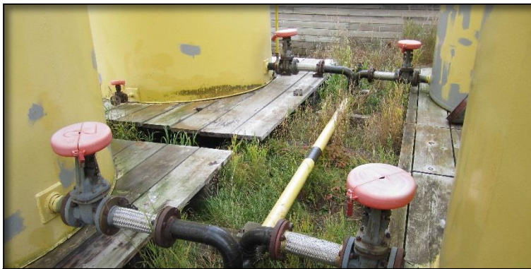
Vegetation Growing in Tank Farm (ADEC 2012)
