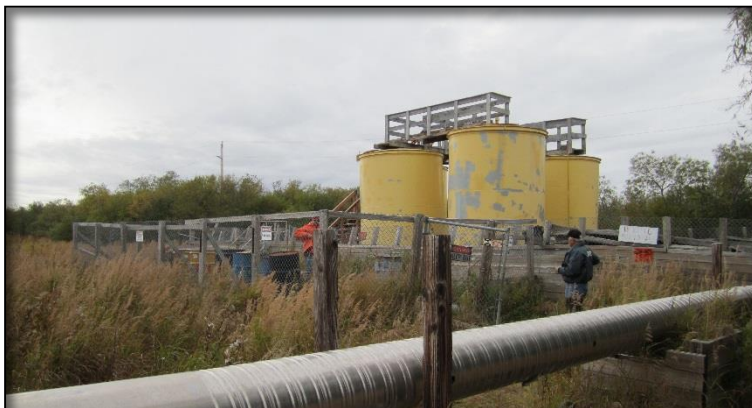
School Tank Farm (ADEC 2012)
