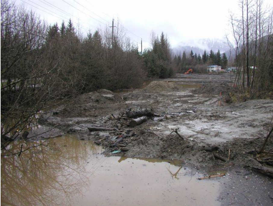
Figure 9a. Photo taken upstream of the Nancy Street bridge and site DC-B on 4/7/06, when sediment was being actively dumped into Duck Creek as part of the wetlands construction project. The activity greatly elevated turbidity and TSS levels downstream.
