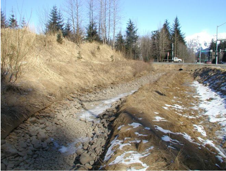
Figure 3a. Site DC-C, showing no flow, on March 15, 2006 when air temperatures reached -15^{\circ}\text{C} in Juneau. No flow was observed at the site for 2 months, from late February to late April, 2006. During this no-flow period, the channel was either completely dry or contained small, stagnant ponds.
