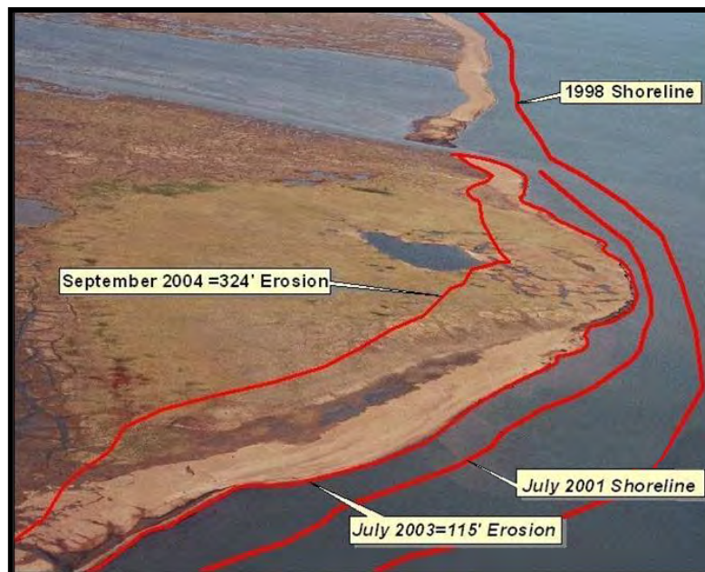
J.W. Dalton Drill Site Erosion. Located east of Barrow on the Beaufort Sea near Teshekpuk Lake and Point Lonely DEW line site. This photograph was taken in 2003 and you can see that between the summers of 2003 and 2004 over 300' of shoreline eroded away along part of the site. Approximately 600' of coastal plain were lost over a six year period. Photo provided by BLM
