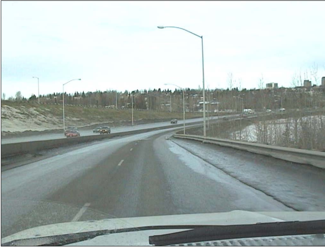
Figure 3(a). Minnesota Drive, March 16, 2000. Ice covers most of roadway margin.
