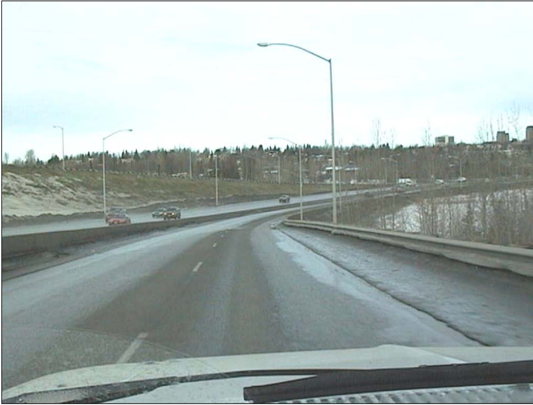
Figure 3(a). Minnesota Drive, March 16, 2000. Ice covers most of roadway margin.
